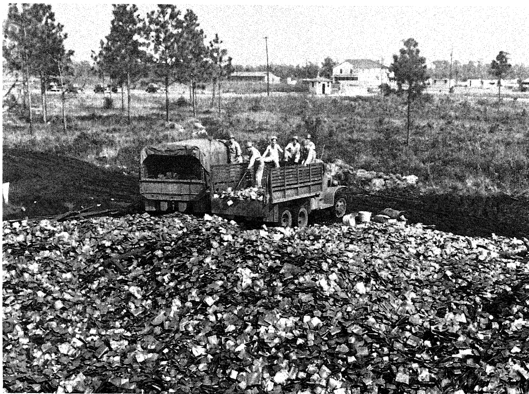
SALVAGE TIN DUMP, Camp Davis, N. C.
