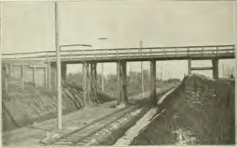
OVERHEAD CROSSING NEAR JULIETTA, INDIANA.
