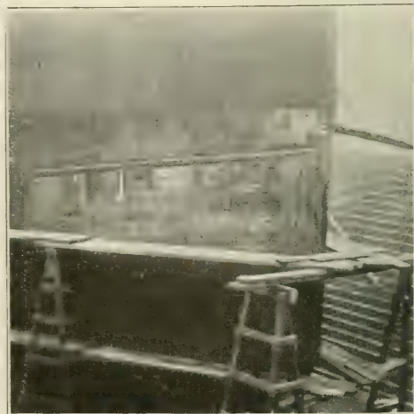
WOODEN TEMPORARY BOW FITTED TO SS. "ROTTERDAM."
