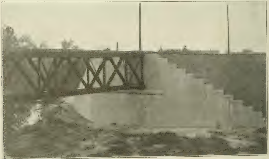
105-FOOT BRIDGE OVER BIG SUGAR CREEK, NEAR PALESTINE, INDIANA.
