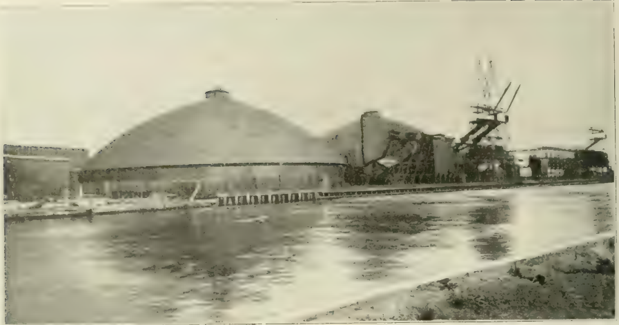
COAL-STORAGE PLANT OF LEHIGH VALLEY COAL COMPANY AT WEST SUPERIOR, WIS. Providing for 100,000 tons of anthracite coal in two circular steel buildings, each 246 feet in diameter and 90 feet high.
