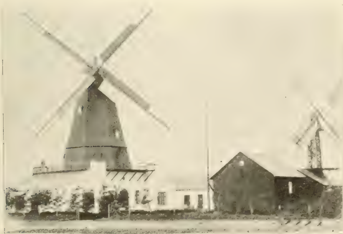
FIG. 1. WIND-DRIVEN ELECTRICAL PLANT AT ASKOV, DENMARK.
