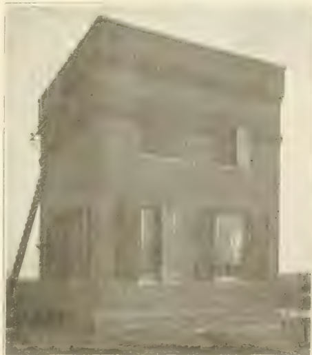
TRANSFORMER STATION AT REEDVILLE, INDIANA.
