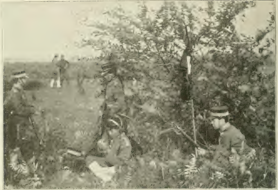
OUTPOST TELEPHONE STATION.
