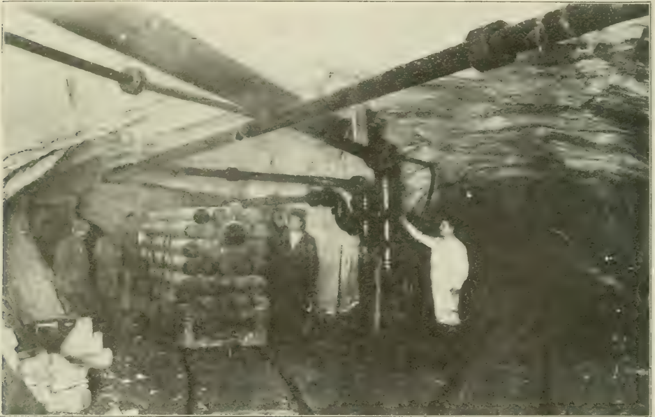
COMPRESSED-AIR LOCOMOTIVE IN TUNNEL.
