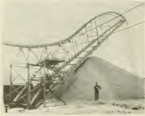
TRIMMER IN OPERATION.
