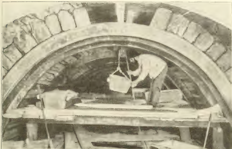
MASONRY ARCHING IN TUNNEL.
