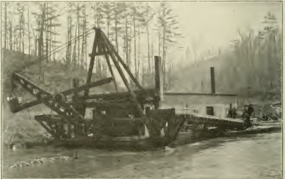
ONE-YARD DREDGE USED IN PLACER MINING AT DAHLONEGA, GEORGIA.
