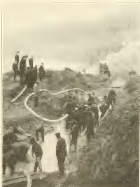
REMOVING RAILROAD OBSTRUCTIONS BY HYDRAULICKING. Illustrating method adopted by Great Northern Railway in the State of Washington, near the coast of Puget Sound, where landslides are continually obstructing tracks.
