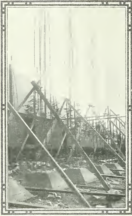
THE STEEL RODS READY FOR THEIR CONCRETE COVERING
