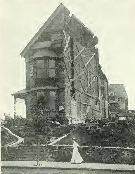
MAKING READY TO MOVE THE LAST SECTION TO THE NEW LOCATION.
