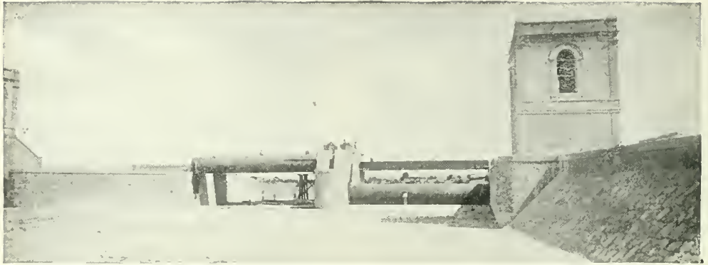
ROLLING DAM IN MEXICO. ONE STEEL CYLINDER LOWERED, THE OTHER RAISED.
