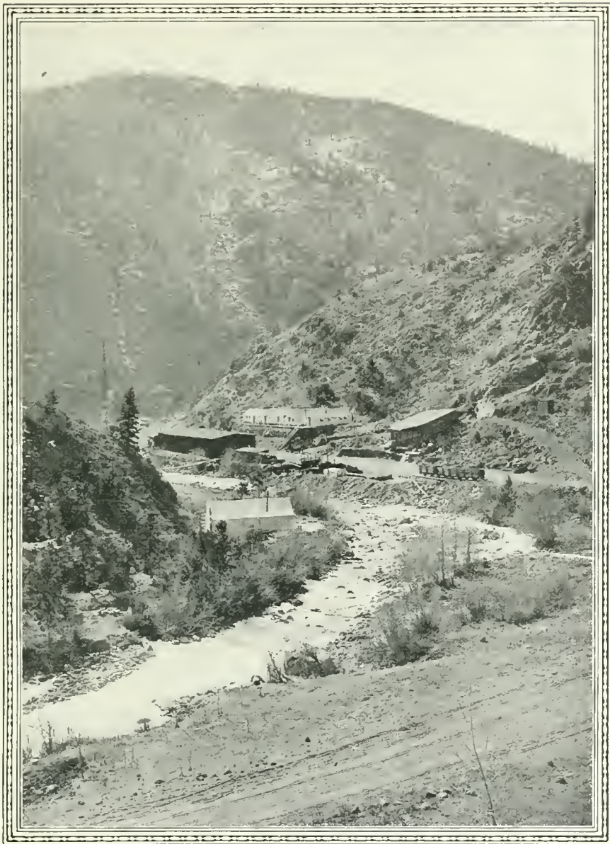
ONE OF THE CAMPS OF THE PIPE LAYERS.
