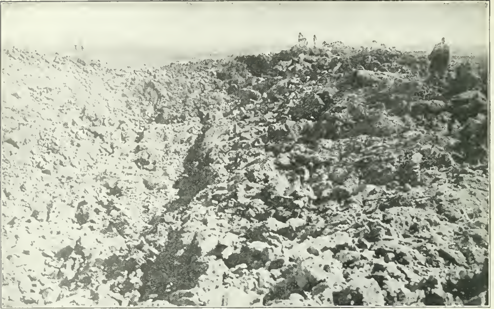
WHAT A THOUSAND TONS OF POWDER AND DYNAMITE CAN DO. This is where the powder mill stood.
