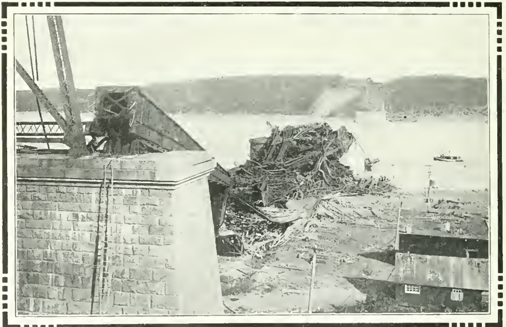
NINE THOUSAND TONS OF STEEL, BENT AND TWISTED INTO INDESCRIBABLE CONFUSION, WHICH HAD TO BE CLEARED AWAY.
