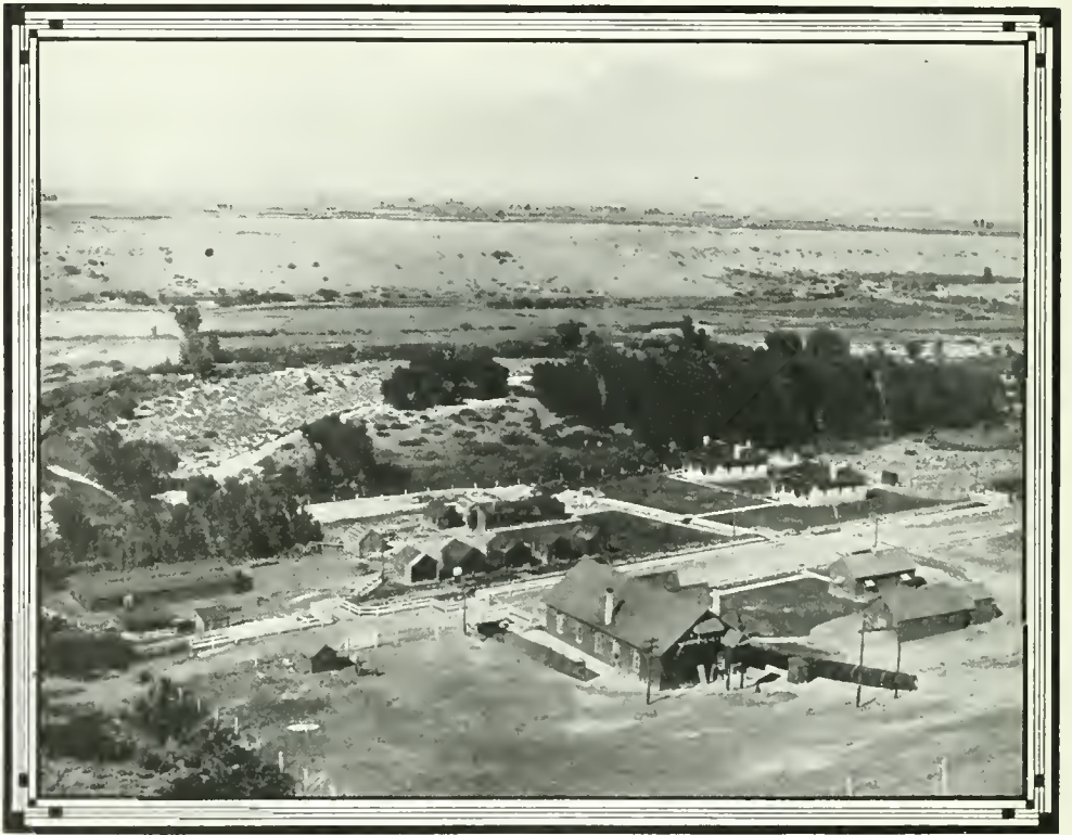
THE UPPER PHOTO SHOWS WHERE THE WATERS OF SPANISH FORK FLOW DOWN THROUGH A PIPE, TO FURNISH POWER. THE LOWER PHOTO SHOWS THIS POWER HOUSE.
