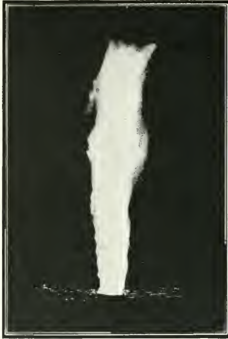
BURNING GAS WELL WITH FLAME 125 FEET HIGH. Photograph taken at night.
