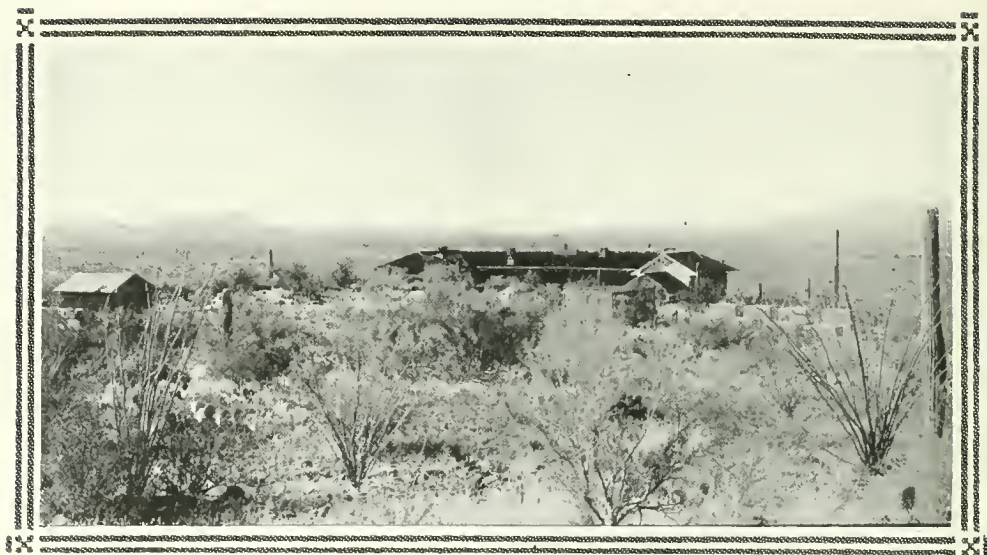
A STATION FOR PLANT STUDY IN THE DESERT. Department of Botanical Research, at Tucson, Arizona.
