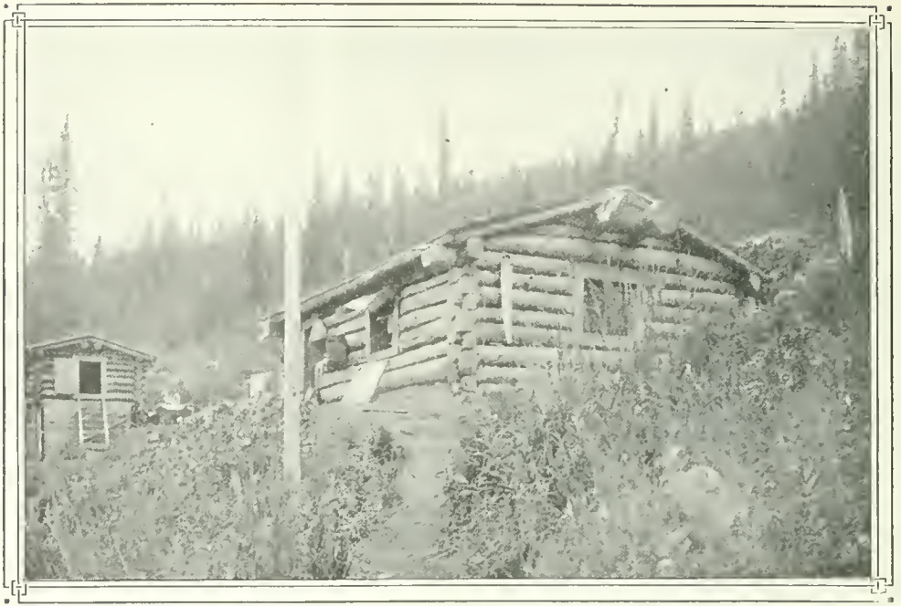
TYPICAL ALASKA TELEGRAPH STATION AND SIGNAL CORPS DETACHMENT QUARTERS, WITH STOREHOUSE FOR SUPPLIES.
