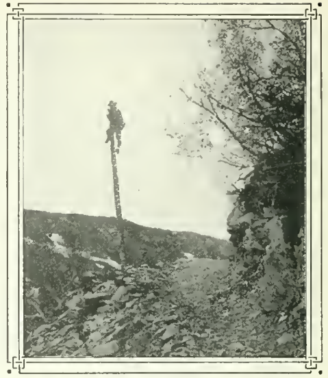
STRINGING A WIRE.
