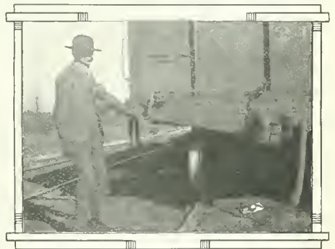
THIS COUPLER RENDERS IT UNNECESSARY TO GO BETWEEN THE CARS. A contrivance that saves hundreds of lives annually.
