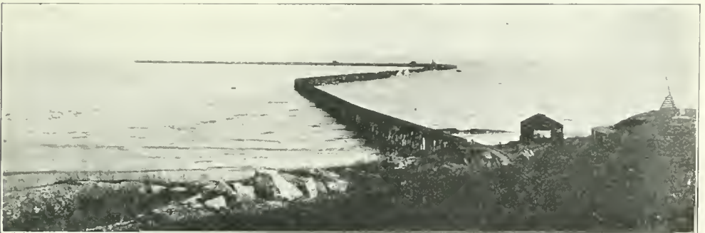
LOS ANGELES' BREAKWATER, WHICH COST $3,000,000 TO BUILD.
