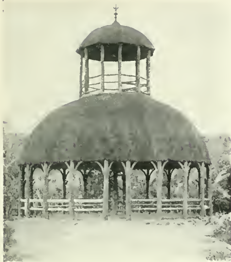
SUMMER HOUSE OF CONCRETE BUILT IN IMITATION OF A STRAW HUT.
