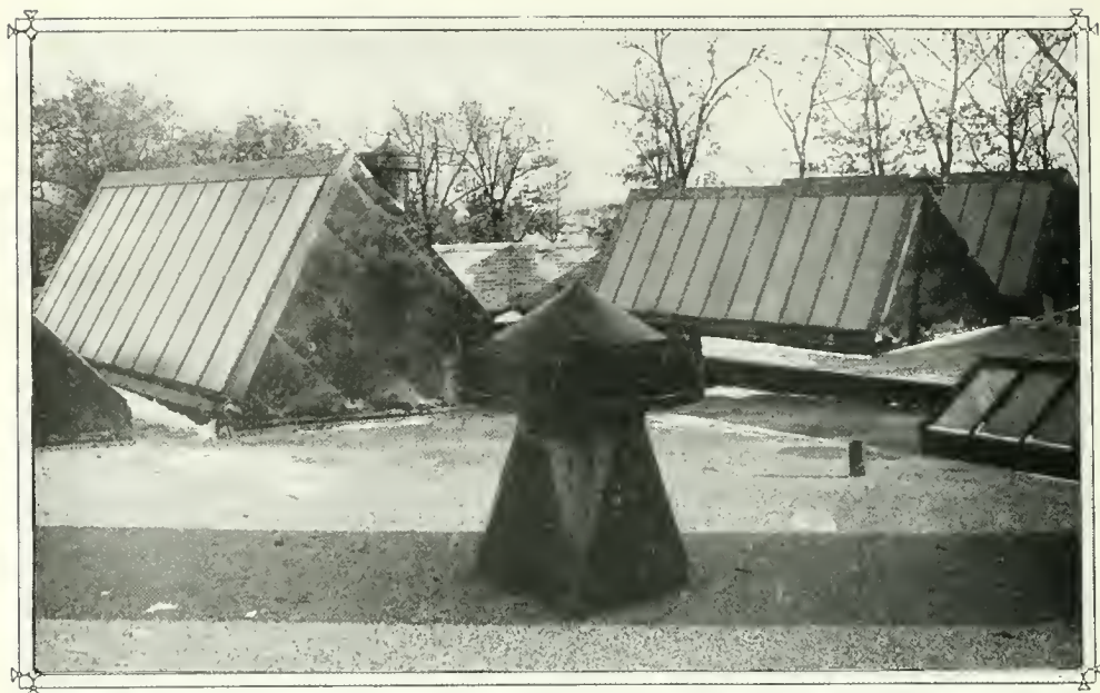
THE SAW-TOOTHED SKYLIGHTS WHICH ARE PARALLEL RIDGES RUNNING EAST AND WEST. The south slope is covered with tin, the north is of reinforced ribbed glass. Thus a steady north light is assured.
