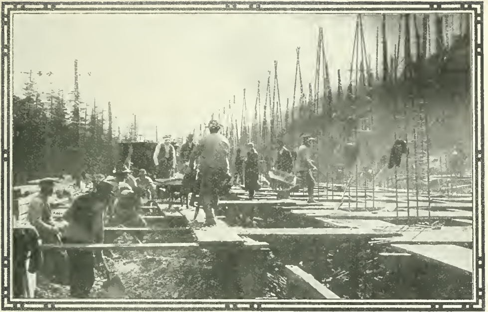
MIXING GRAVEL AND CEMENT FOR THE CONCRETE SNOWSHEDS IN THE CASCADE MOUNTAINS.
