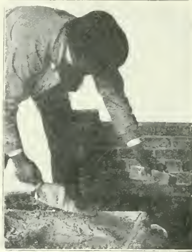
IN LAYING BRICKS APPRENTICES SHOULD BE TAUGHT TO USE BOTH HANDS AT ONE TIME.
