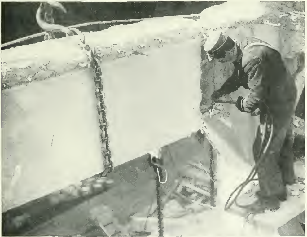
CUTTING A GIRDER IN TWO WITH A BLOW PIPE. The workman has a most limited space for footing.
