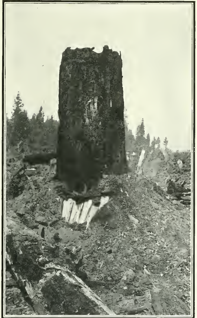
THE FUEL IN PLACE, READY FOR FIRING.
