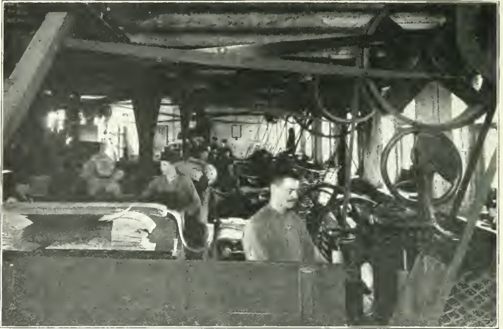
THE PEELING OR VENEERING ROOM OF A MATCH FACTORY.
