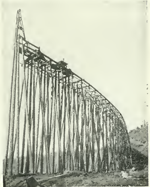
ONE OF THE LAST OF THE WOODEN TRETTLES. This is over a small stream in California. Steel is rapidly replacing such bridges as this.
