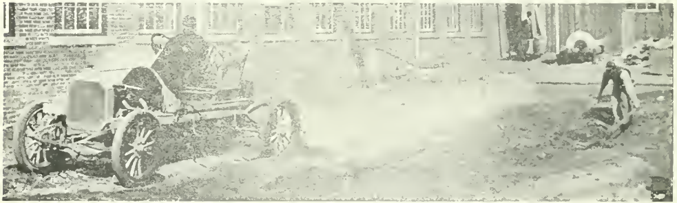
EQUAL TO SIX TEAMS OF HORSES. Automobile which proved its efficiency by excavating for a 5,000 gallon gasoline tank. There seems to be no end to the uses to which this pleasure machine may be put.
