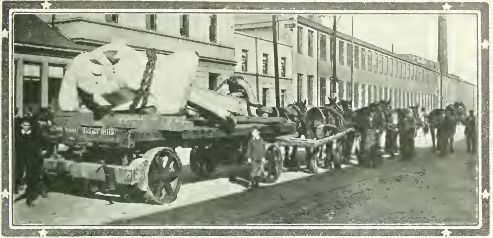
DELIVERING ONE OF THE FIFTEEN TON ANCHORS.
