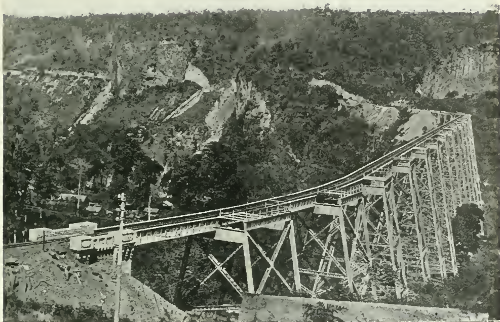
DARING SWEEP IN BURMAH'S FAMOUS BRIDGE. At the curve is a silver bolt which was the last bolt used in the work.
