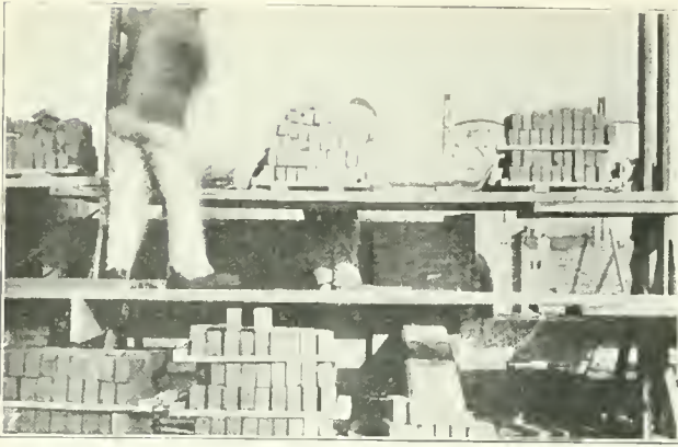
THE NON-STOOPING SCAFFOLD.
