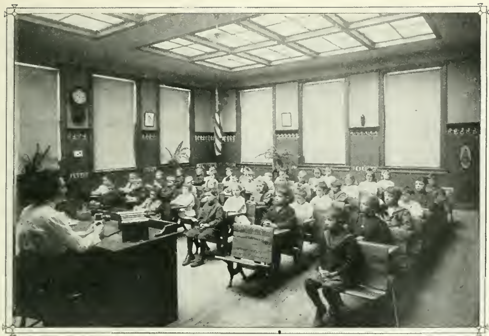
THE ONLY WAY TO SECURE A WELL-DISTRIBUTED LIGHT IS FROM OVERHEAD. This illustration shows a room in the new sky lighted school in River Forest.
