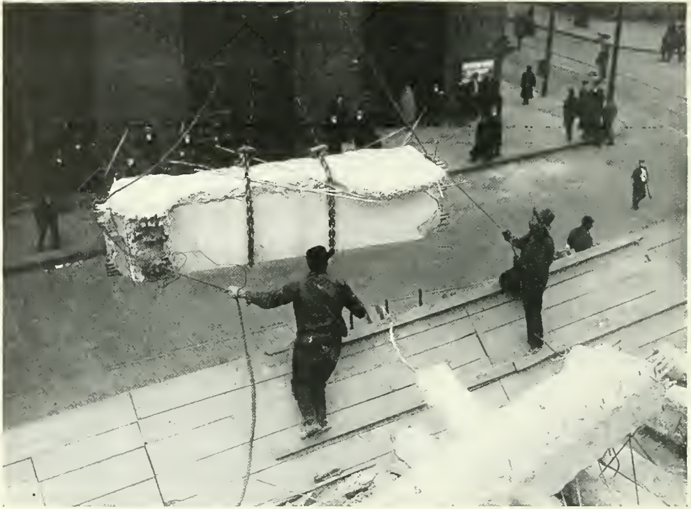
LOWERING A CONCRETE GIRDER.
