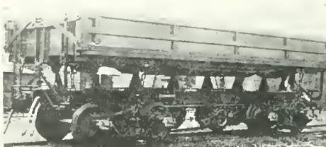
PANAMA CANAL DUMP CAR AS IT APPEARS LOADED.
