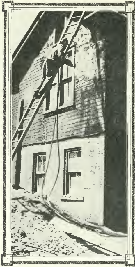
APPLYING CEMENT STUCCO TO AN OLD BUILDING AFTER COVERING IT WITH WIRE MESH.
