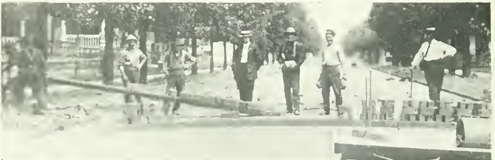
ROLLER BRICK CARRIER BANISHES THE WHEELBARROW.
