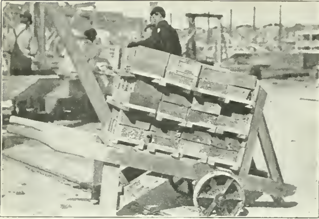
THE BEST METHOD, UP TO DATE, FOR HANDLING BRICK. This barrow holds 216 bricks as against the usual 60.
