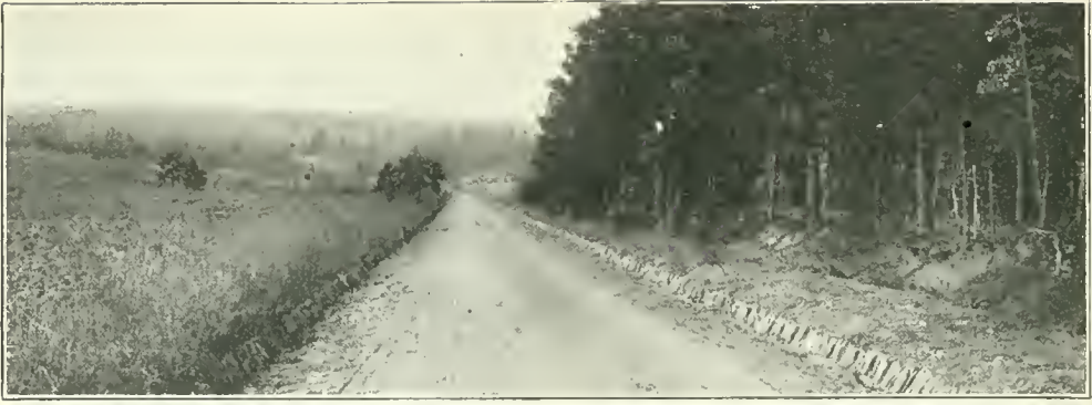
AUTOMOBILES TEAR TO PIECES ROADS LIKE THIS. A macadam road in Georgia.
