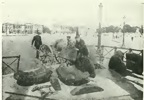
PUTTING TOGETHER THE HOLLOW WOODEN BALL FOR CLEANING PARIS' SEWERS.
