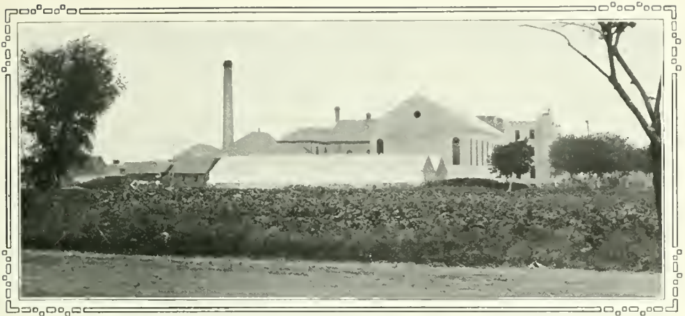
GREENHOUSE AND OTHER BUILDINGS HEATED AND LIGHTED WITH STEAM AND ELECTRICITY GENERATED FROM THE BURNING OF GARBAGE.
