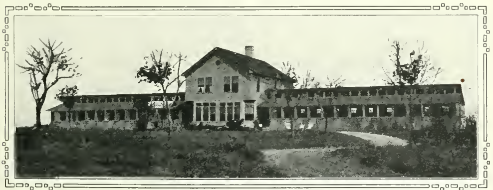
HOPEWELL TUBERCULOSIS HOSPITAL, HEATED AND LIGHTED BY THE CREMATORY PLANT.
