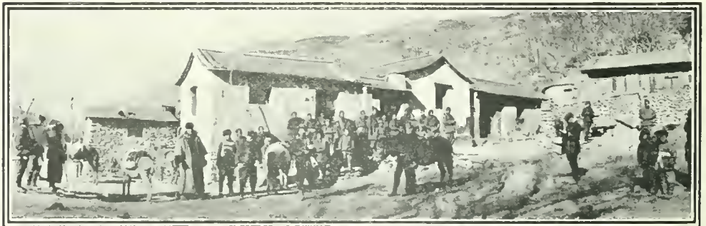
SUPERVISING THE CONSTRUCTION OF THE CABLEWAY. The arrival at Nantziou.
