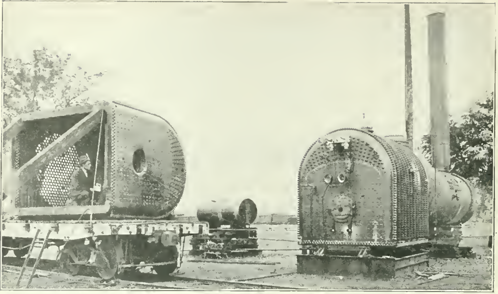
AN ENGINEER MADE RECORDS OF THE TEST FROM THE INTERIOR OF A FIREBOX CHAINED TO A FLAT CAR A SHORT DISTANCE FROM THE BOILER.
