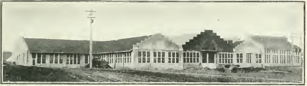
FACTORY AT MOSCOW, IDAHO, WHERE THE NEW HARVESTER IS MANUFACTURED. The buildings are of concrete, stone and glass.
