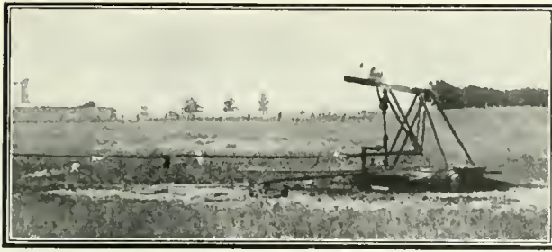
JACK USED IN PUMPING OIL FROM A WELL.
