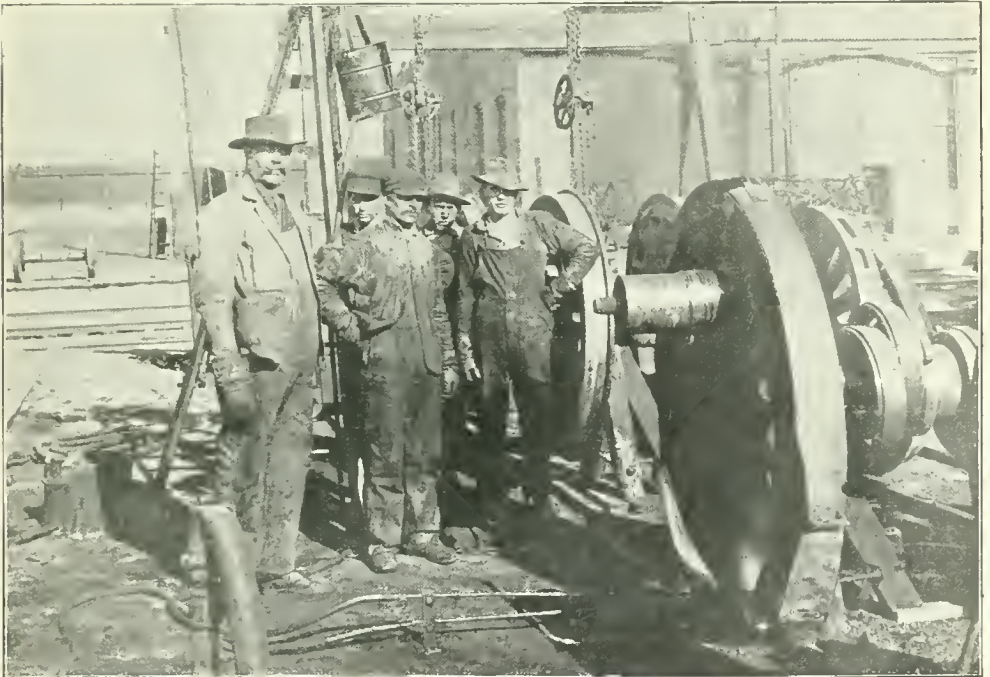
APPARATUS USING CRUDE OIL IN PLACING AND REMOVING TIRES. Note how the hot flame is directly applied to the tire.
