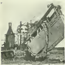
DIGGING TILE DITCH TO RECLAIM LAND.
