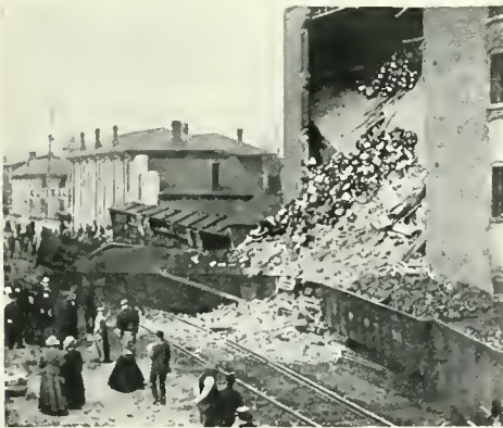
BRICK BUILDING DEMOLISHED BY A STEEL COAL CAR.
