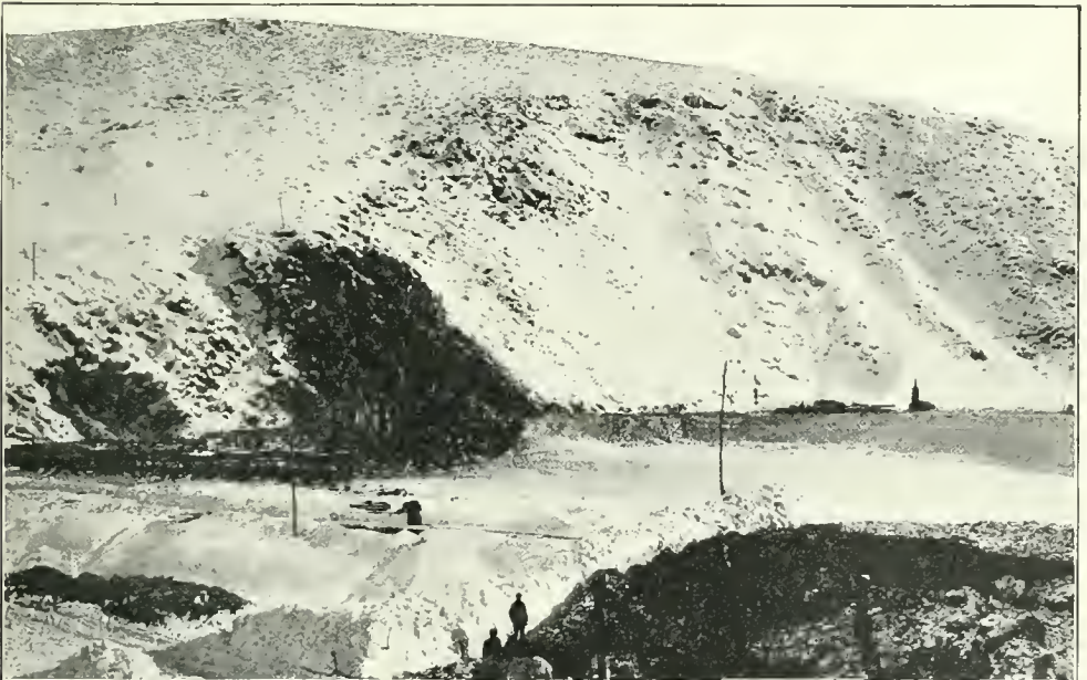
THE EXCAVATION WORK IN THE HILLSIDE, WHERE, LATER, ROCK WAS SET INTO ROCK. View of the gorge at the dam site.
