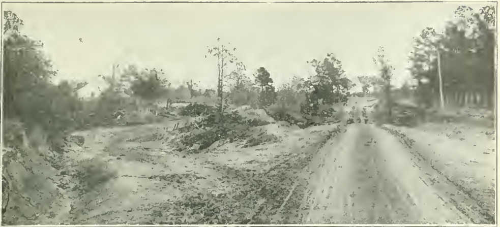
AN OBJECT LESSON OF THE UNITED STATES OFFICE OF PUBLIC ROADS, AT MONROE, I.A. The old highway to the left, and the new.
