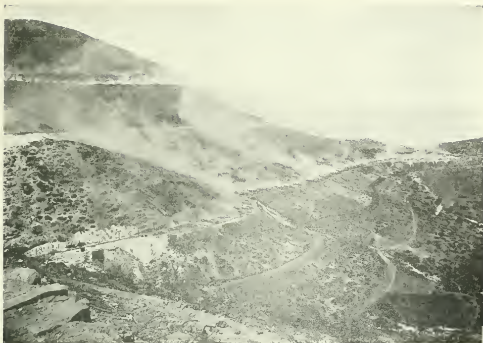
ROASTING COPPER ORE ON A GIGANTIC SCALE AT JEROME, ARIZONA.
