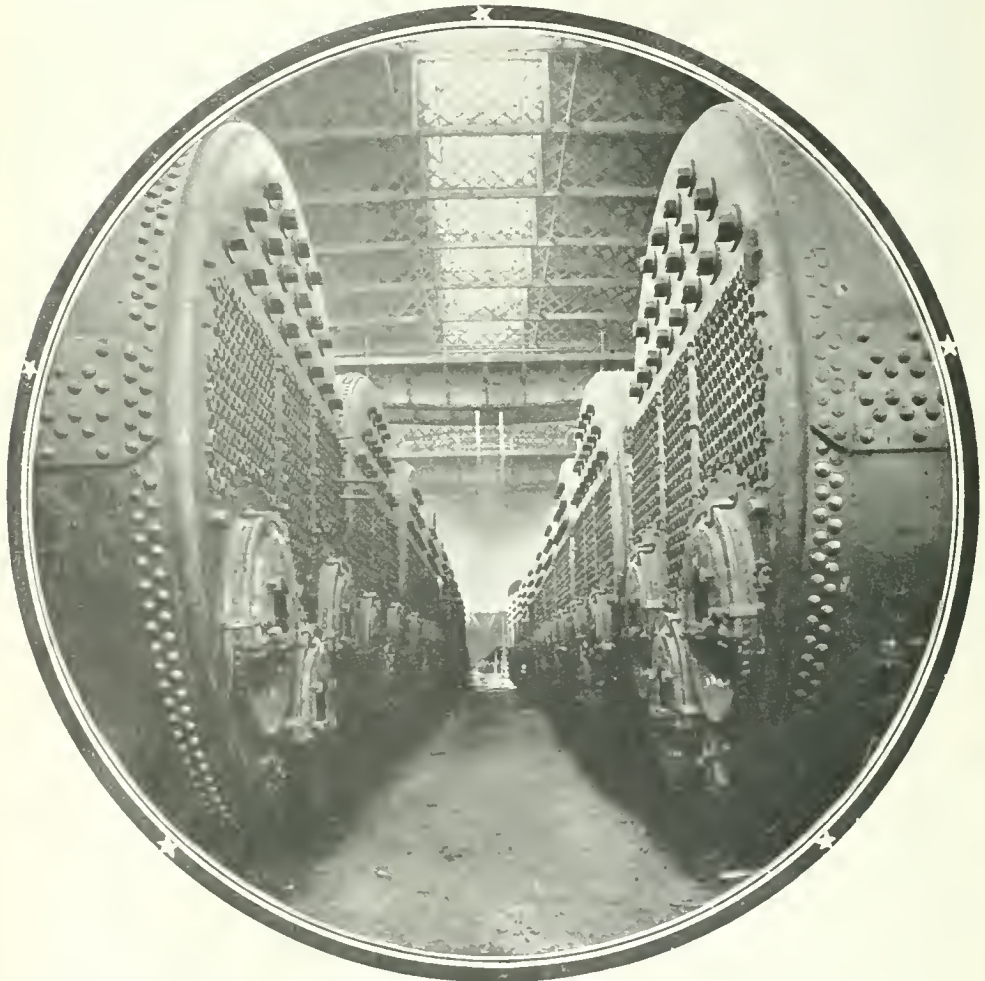
ALL PARTS OF THE VESSEL ARE GIGANTIC. The boilers are 15 feet, 9 inches in diameter and 20 feet in length.
