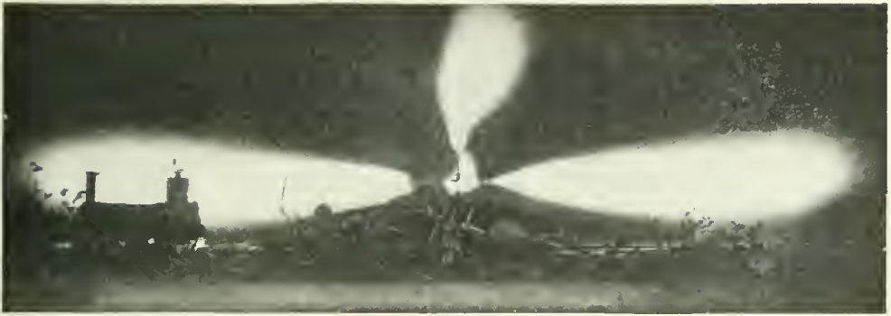
GAS WELL ON FIRE NEAR HAMBURG, GERMANY. The outburst could not be checked, and had to be fired to purify the atmosphere.
