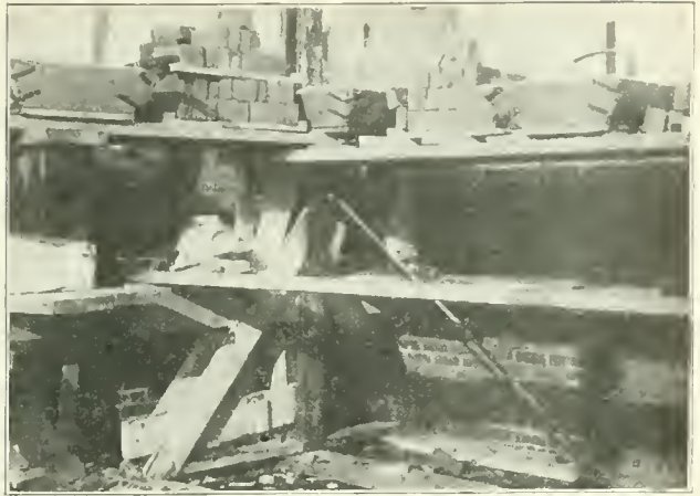
NON-STOOPING SCAFFOLD WITH BRICKS SYSTEMATICALLY SET UP IN A CORNER.
