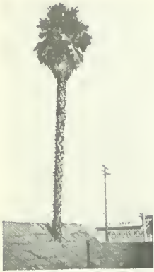
PALM TREE GROWING THROUGH ROOF. A 60-foot curiosity of Los Angeles, that is due to owner's sentimentality.
