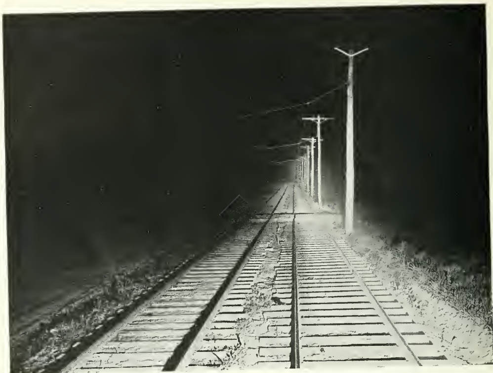
THIS PHOTO WAS TAKEN BY THE RAYS OF AN INTERURBAN ELECTRIC CAR LIGHT. The arc lamp is about fifteen inches in diameter and nine inches in depth. It illuminates for five hundred yards.
