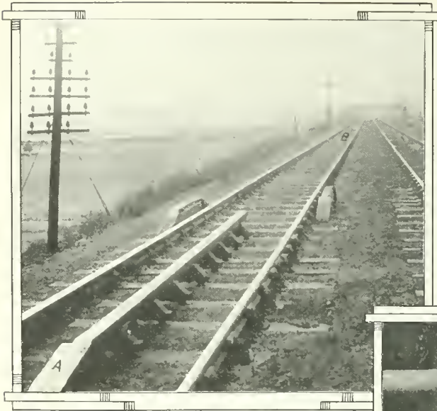
CONTACT RAIL, WHICH TOUTS THE WHISTLE OF THE PASSING LOCOMOTIVE WHEN DANGER THREATENS.
