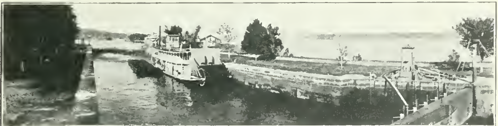
THREE LOCKS, SIMILAR TO THIS, IN OPERATION FORTY YEARS, WILL BE COMPLETELY SUBMERGED.
