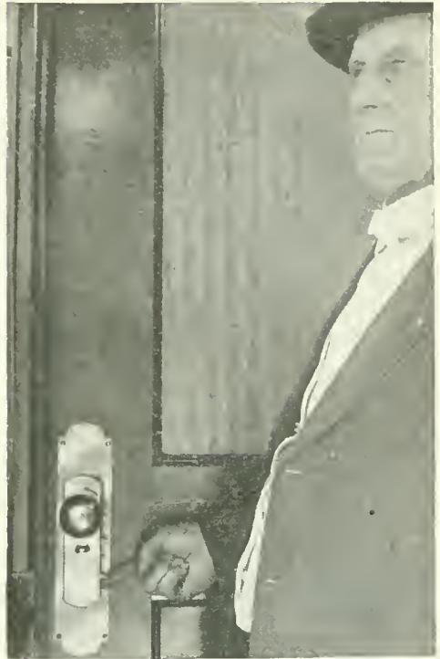
A KEYLESS LOCK THAT IS OPERATED AFTER THE MANNER OF A SAFE COMBINATION.
