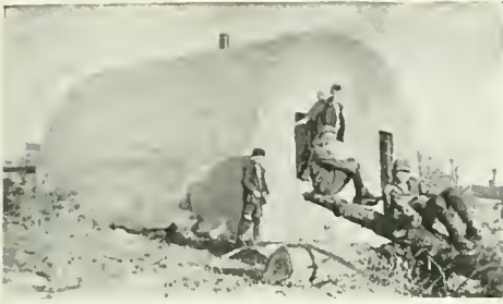
A "JUG" IN NAME AND FACT. This city jail—of concrete—at Mansfield, Mo., is, however seldom used.
