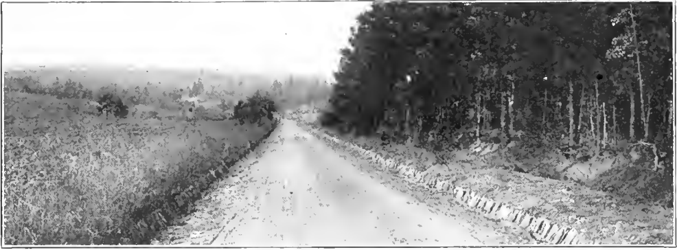
AUTOMOBILES TEAR TO PIECES ROADS LIKE THIS. A macadam road in Georgia.
