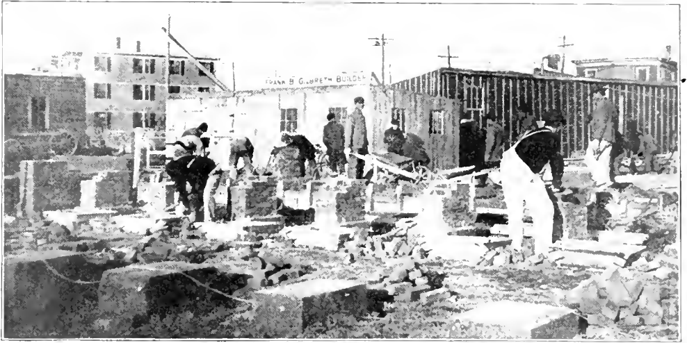
THE WRONG WAY OF LAYING OUT THE BRICK FOR THE WORKMEN'S USE.
