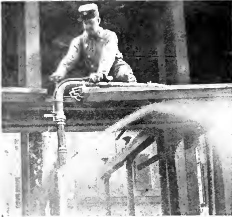
NEW AID TO FIGHT FIRE. An unusual type of deluge pipe.
