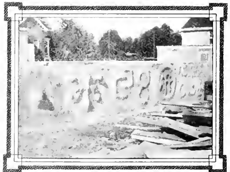
WHAT MAY BE DONE IN BUILDING OUT WITH ONE APPLICATION OF THE CEMENT GUN.
