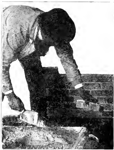
IN LAYING BRICKS, APPRENTICES SHOULD BE TAUGHT TO USE BOTH HANDS AT ONE TIME.
