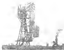
THE CRANE ON THE WATER. This monster is capable of lifting two hundred tons.
