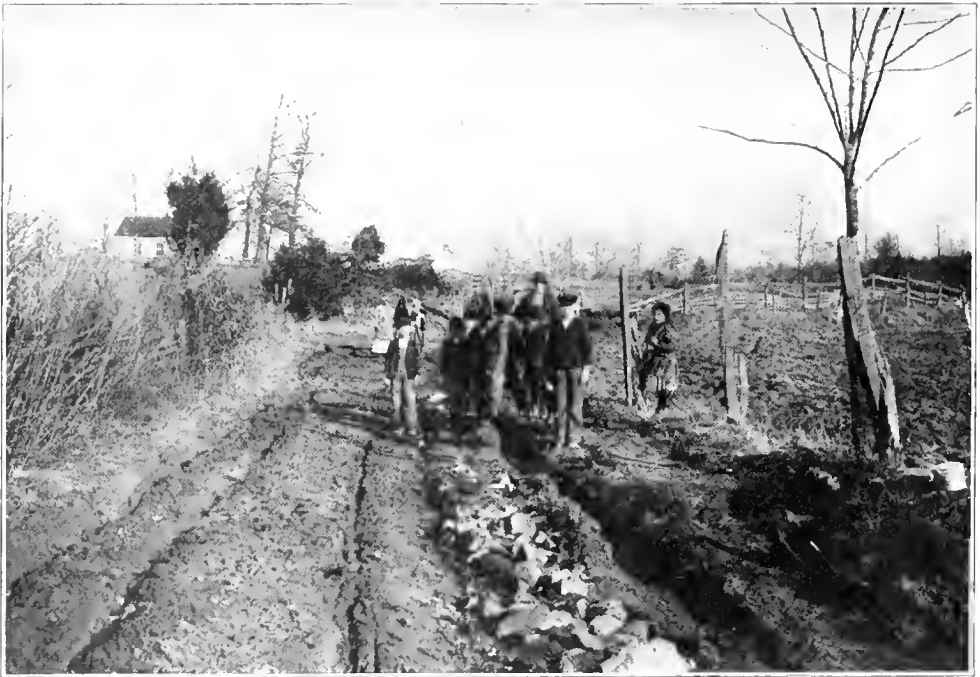
A SCHOOL BUILDING AND A COUNTRY ROAD THAT ANY COMMUNITY SHOULD BE ASHAMED OF.
