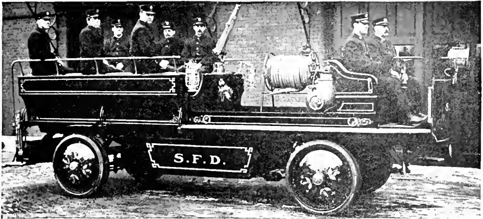
COMBINATION HOSE AND CHEMICAL AUTO USED BY THE SPRINGFIELD, MASS., FIRE DEPARTMENT.
