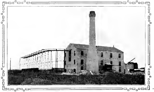
THE CREMATORY BUILDING AND STEEL RUNWAY FOR BRINGING UP THE GARBAGE
