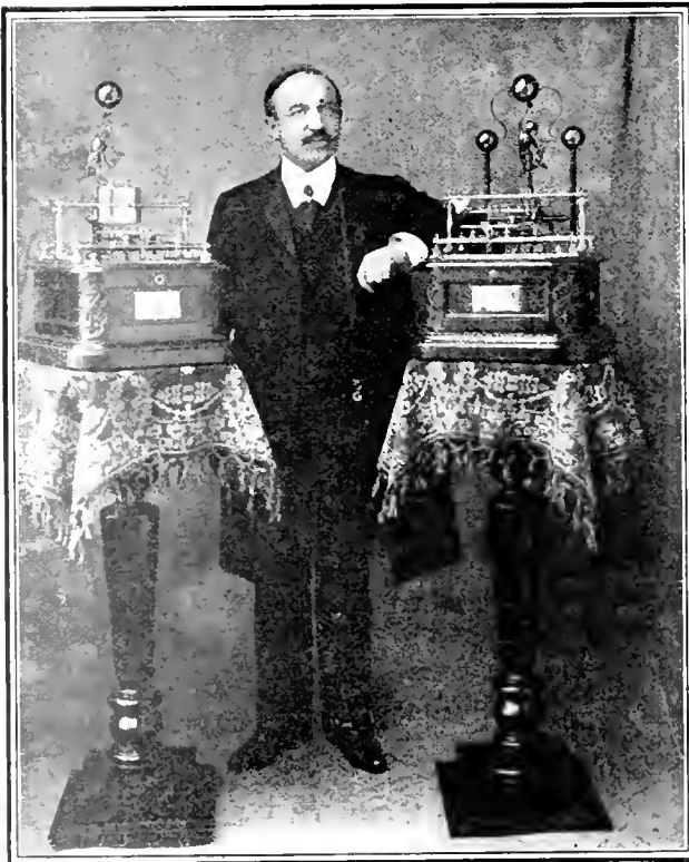
APPARATUS FOR SENDING—REPRODUCING—PICTURES BY WIRELESS. The transmitting machine is at right, receiver at left of the inventor, HANS KNUDSEN.
