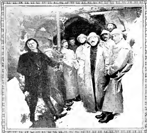
ENGINEERS AND SOME OF THE WORKMEN WHO WERE INSTRUMENTAL IN CONSTRUCTING THE "STRONGEST PIPE."
