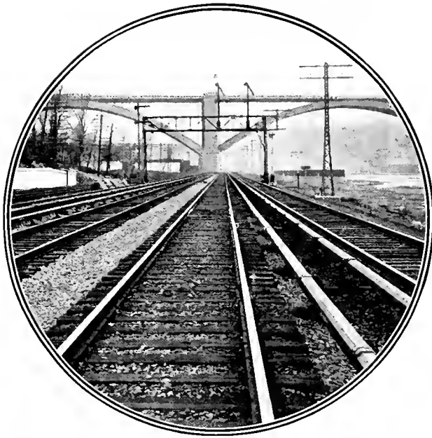
TYPICAL SECTION, SHOWING THIRD RAIL, TRANSMISSION LINE, AND SIGNAL BRIDGE OF ELECTRIFIED PORTION OF THE NEW YORK CENTRAL AND HUDSON RIVER RAILROAD.
