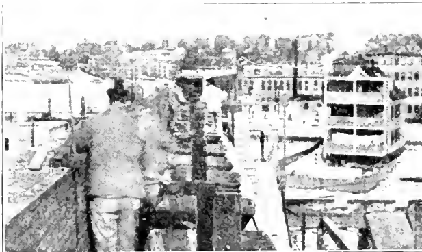
MASONS FINISHING A WALL ON A NON-SLOPING SCAFFOLD.
