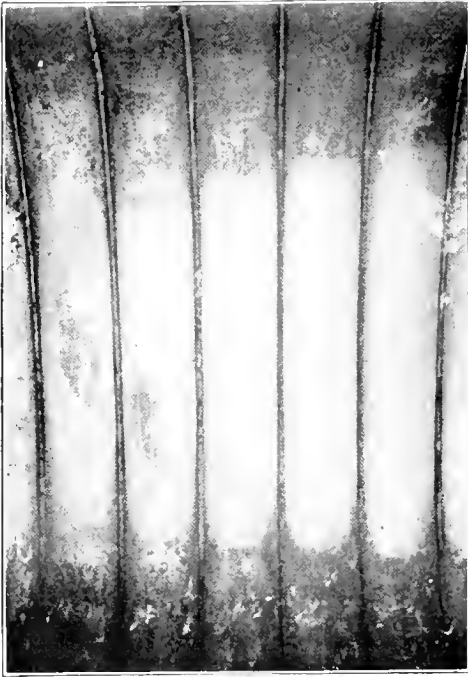
THE INTERIOR OF THE FIREBOX AFTER THE EXPERIMENT SHOWING THE EFFECTS OF THE INTENSE HEAT TO WHICH IT WAS SUBJECTED.
