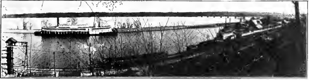
THIS NINE-MILE CANAL, BUILT AT A COST OF $8,000,000, WILL, WITH ITS LOCKS, BE SUBMERGED TWENTY FEET BY THE BACK WATER OF THE DAM.
