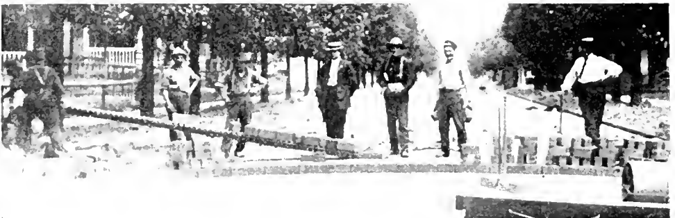
ROLLER BRICK CARRIER BANISHES THE WHEELBARROW.
