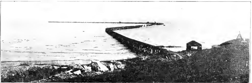
LOS ANGELES' BREAKWATER, WHICH COST $3,000,000 TO BUILD.
