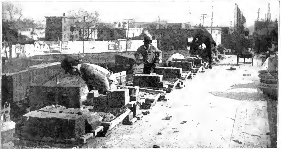
THE RIGHT WAY—IMPROVED METHOD OF HAVING THE BRICKS ON PACKETS AND THE BOXES PROPERLY SPACED FOR THE GREATEST SPEED WHEN THE WALL IS AT THIS LEVEL.
