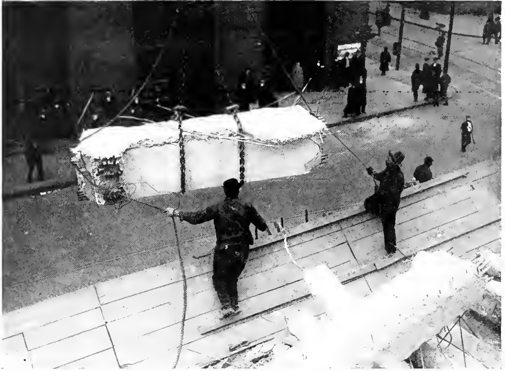
LOWERING A CONCRETE GIRDER.
