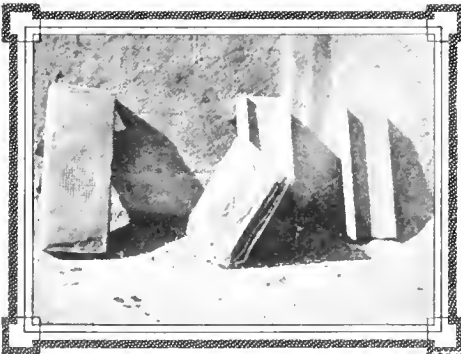
PIECES OF STEEL BEAMS COATED WITH CEMENT SAND MORTAR FOR PROTECTION AGAINST RUST OR CORROSION.
