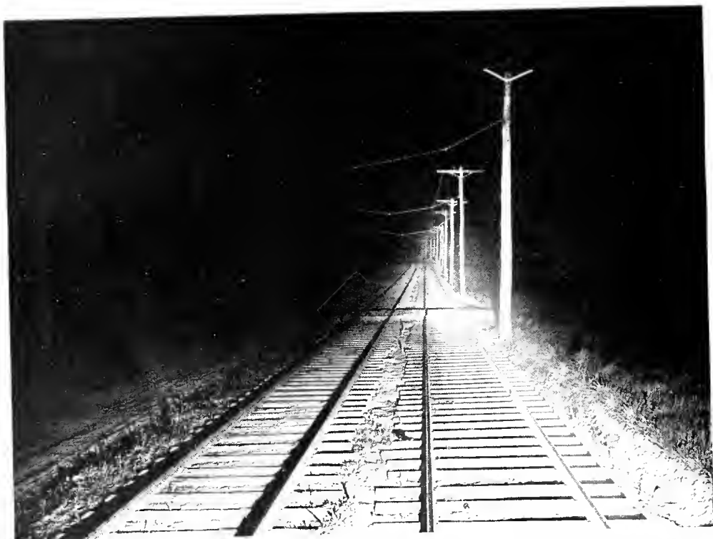
THIS PHOTO WAS TAKEN BY THE RAYS OF AN INTERURBAN ELECTRIC CAR LIGHT. The arc lamp is about fifty inches in diameter and nine inches in depth. It illuminates for five hundred yards.
