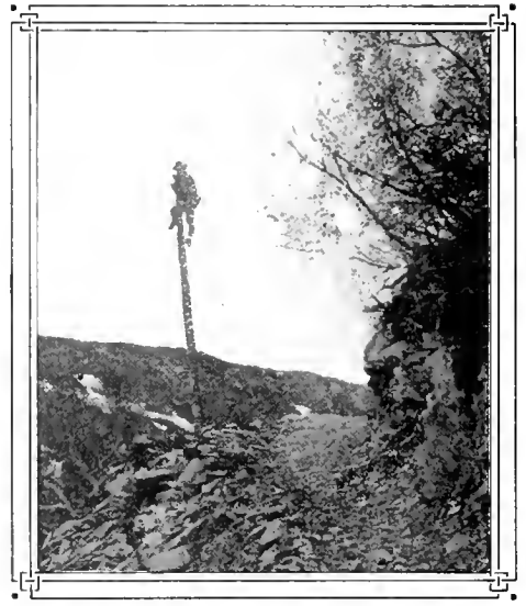
STRINGING A WIRE.
