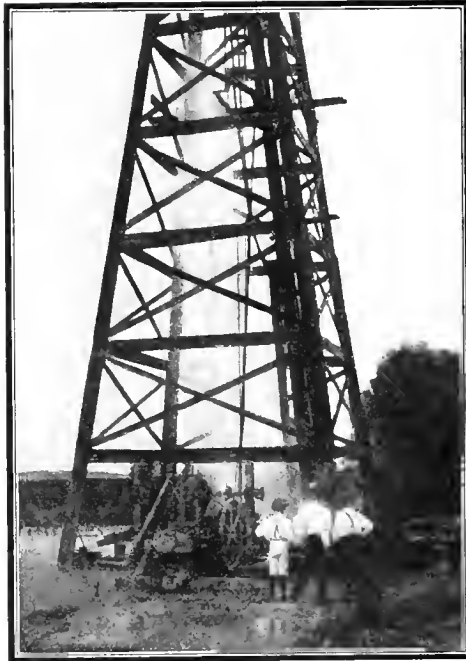
A GAS WELL BEFORE BEING SHUT IN. Where the flow is very strong, the gas usually yields but little gasoline.
