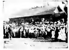
CHURCH BUILT IN SEVEN HOURS. The finished structure and its builders.
