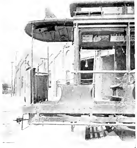
FENDER IN POSITION TO PICK UP A PERSON
