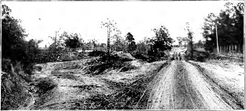
AN OBJECT LESSON OF THE UNITED STATES OFFICE OF PUBLIC ROADS, AT MONROE, LA. The old highway to the left, and the new.
