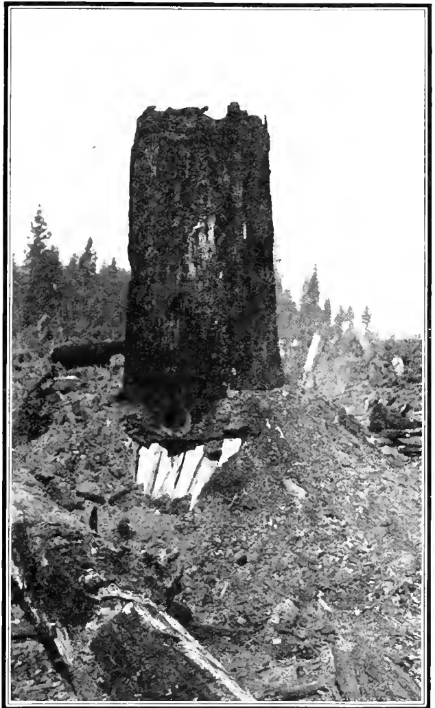
THE FUEL IN PLACE, READY FOR FIRING.
