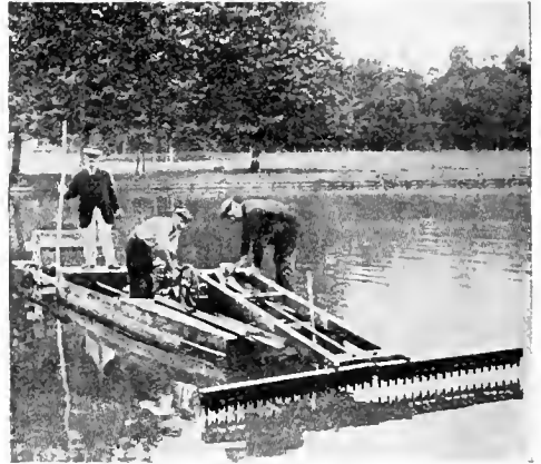
FIG. 2—REPLACING THE APPARATUS IN POSITION
