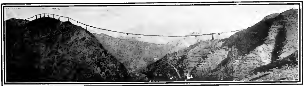
THE NEW METHOD OF TRANSPORTING COAL. Cableway through the Chang-Fan-Chan Mountains, China.
