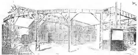
SECTION IN TRAVELING CRANE
