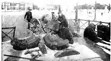
PUTTING TOGETHER THE HOLLOW WOODEN BALL FOR CLEANING PARIS' SEWERS.
