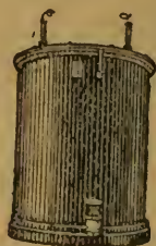
The First 10,000 Volt Transformer
