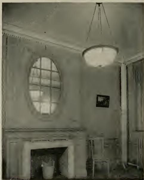
INDIRECT BOWL FOR HOUSE LIGHTING—MULTIPLE NITROGEN LAMP
