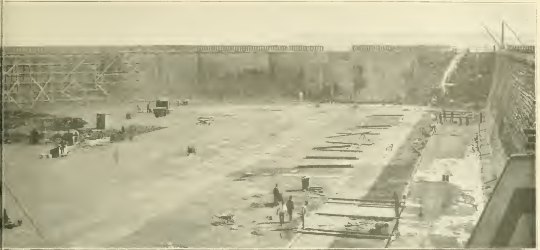
dry stage of the work of waterproofing floor and walls
