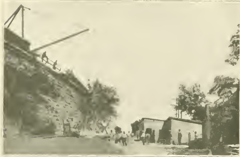
Fig. 6. Cement Gun Contractors Plant
