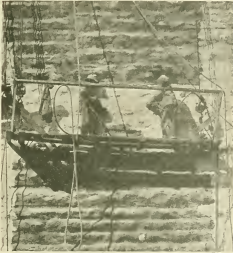
Fig. 3. Part of Basin Wall showing method of removing asphalt coating
