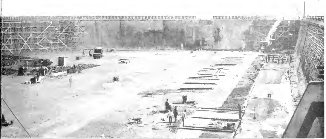
Every stage of the work of waterproofing floor and walls
