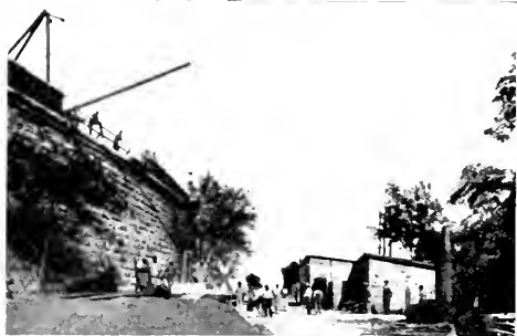
Fig. 6. Cement Gun Contractors Plant
