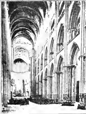
FIG. 3. INTERIOR OF CATHEDRAL AT ROUEN
