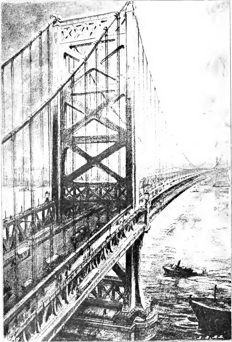
THE DELAWARE RIVER BRIDGE
