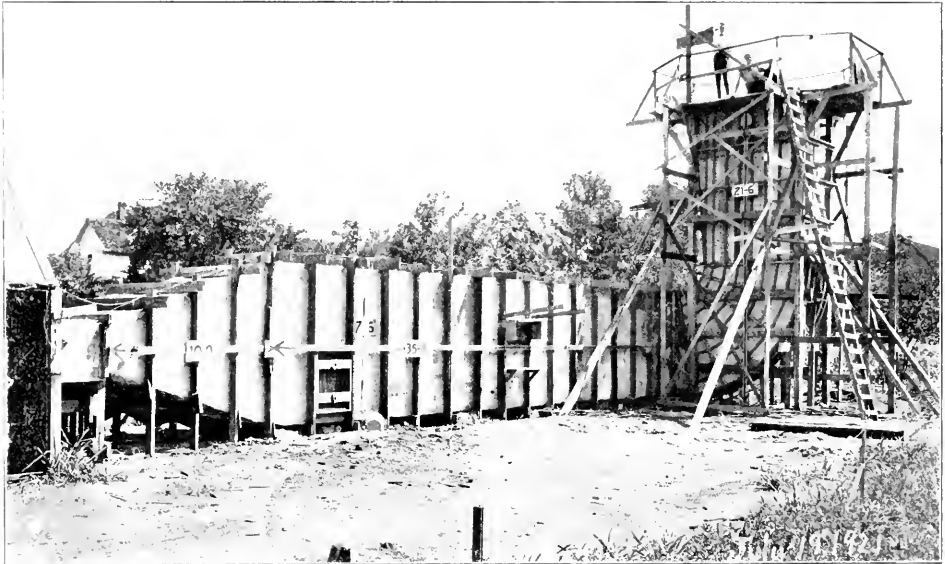
FIG. 17. LARGE SIZE COMPOUND ELBOW MADE OF CONCRETE.
