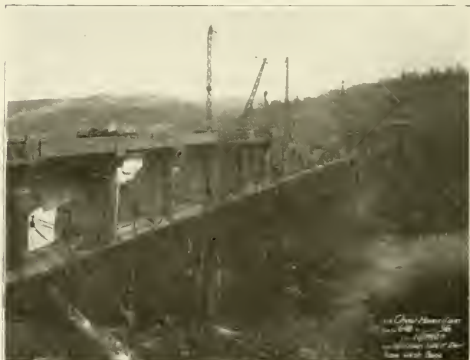
Figure 5—UPSTREAM SIDE OF DAM
