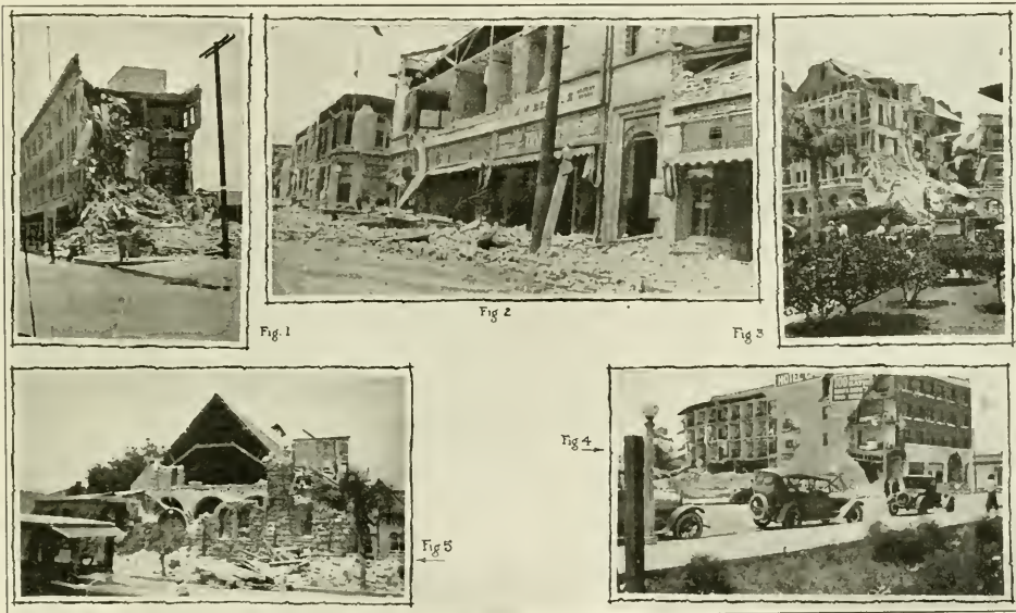
VIEWS OF DESTRUCTION CAUSED BY SANTA BARBARA EARTHQUAKE
