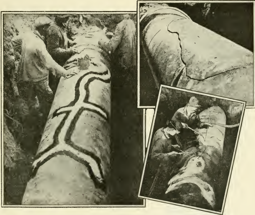
FIGURE 4.—ILLUSTRATIONS SHOW HOW TOBIN BRONZE WELDING RODS WERE USED TO SEAL A 13 FT. FRACTURE IN A WATER MAIN AT WASHINGTON, D. C. (Photo by Courtesy of American Brass Company.)
