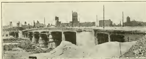
FIG. 4 THE 23RD STREET VIADUCT
