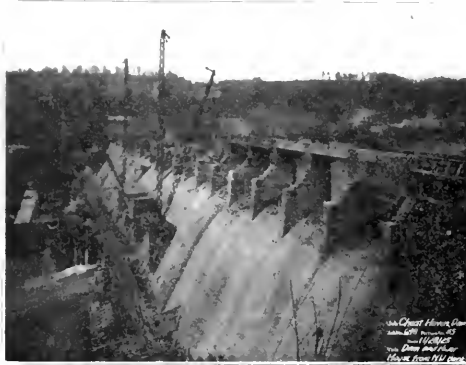
Figure 1—DAM AND POWER HOUSE
