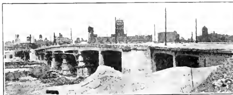
FIG. 4 THE 23RD STREET VIADUCT
