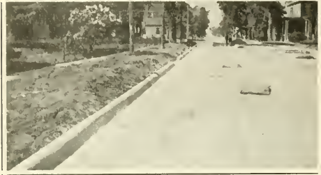
Curing with Calcium Chloride
