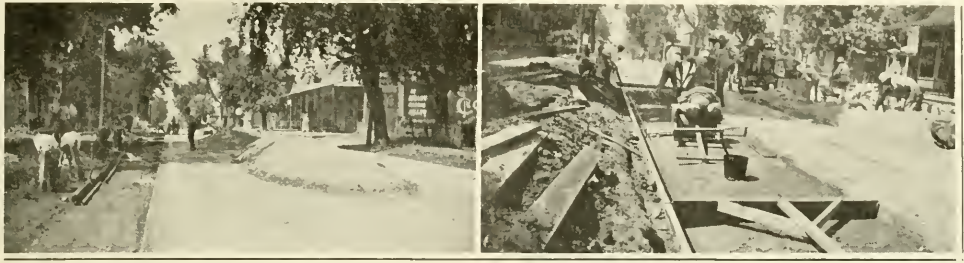
Setting Forms and Preparing Subgrade for Pouring
