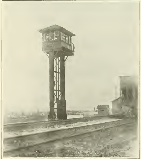
Switch Operator Tower
