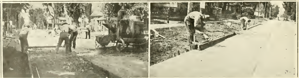
Pouring Concrete and Building Integral Curb
