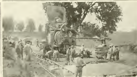
Fig. 9—Mixer in operation
