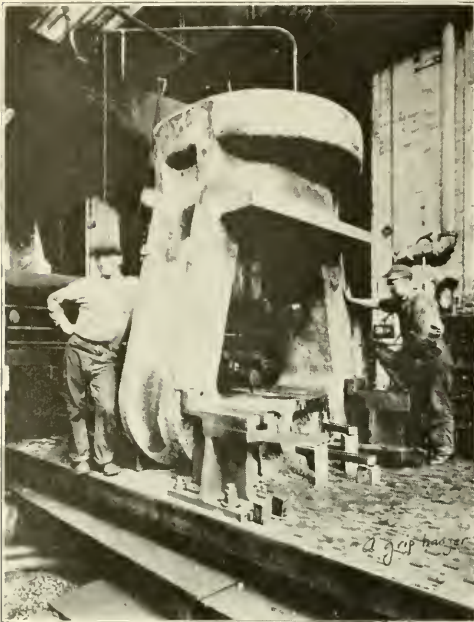
Machining Pulling Head of 3,000,000 Pound Testing Machine
