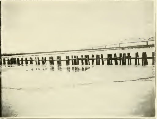
Fig. 4. A Standard Pile Clump Dike
