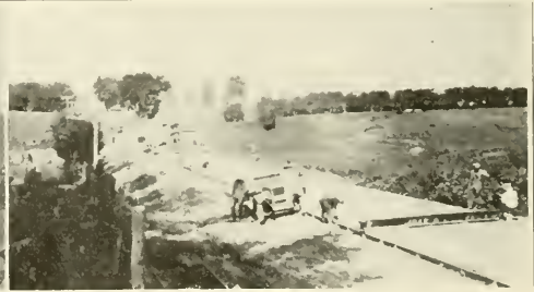
Fig. 10—Concrete being dumped on subgrade
