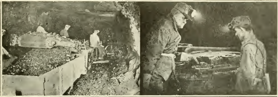
Loading a car with a machine loader
