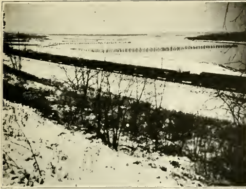
Fig. 2. Dikes Used to Throw the Channel Back
