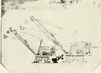
A comparison: the big shovel; the previous record size; and, in solid black, the standard-size excavating shovel
