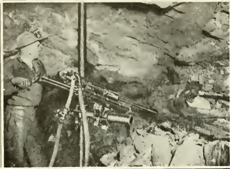
Drifting in a copper mine
