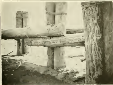
Fig. 4. Revetment for Bank Protection
