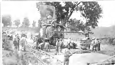
Fig. 9—Mixer in operation
