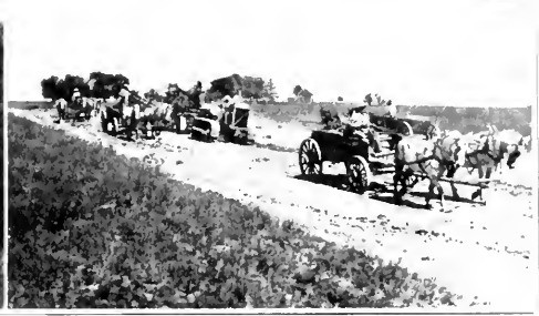
Fig. 4—Thirteen foot cut at start of excavation
