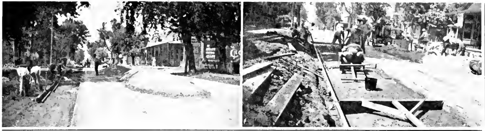
Setting Forms and Preparing Subgrade for Pouring
