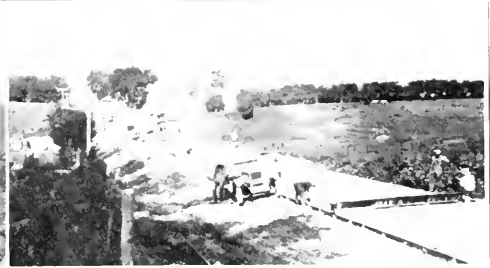
Fig. 10—Concrete being Dumped on subgrade
