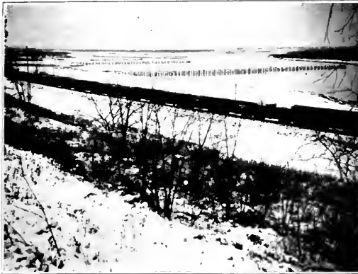
Fig. 2. Dikes Used to Throw the Channel Back
