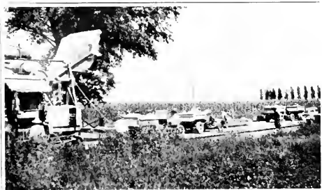
View showing mixer and trucks at work
