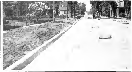
Curing with Calcium Chloride
