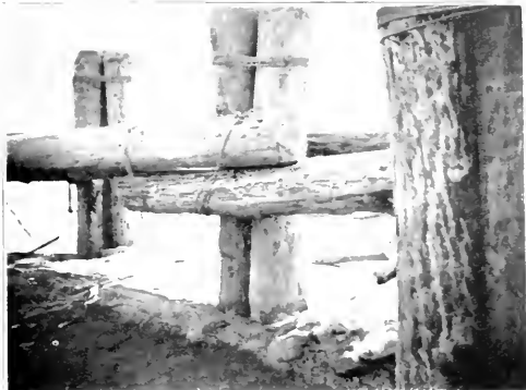
Fig. 4. Revetment for Bank Protection.
