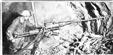
Drifting in a copper mine
