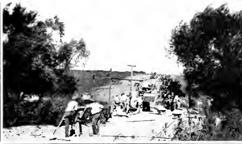
Fig. 2—Box culvert at Station 4-15
