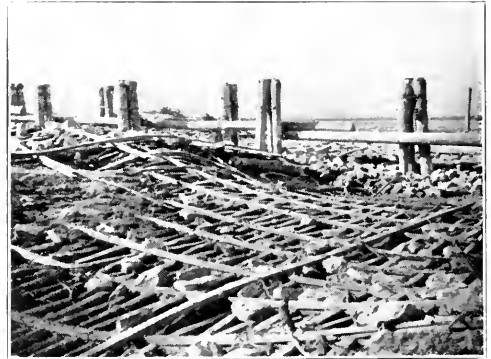
Fig. 6. Mat Laid on River-Bed Revetment for Bank Protection
