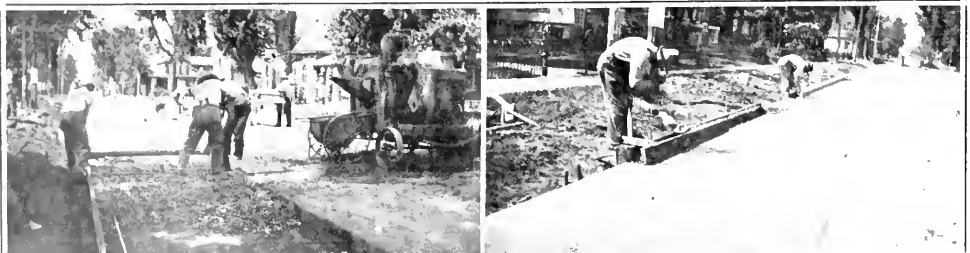
Pouring Concrete and Building Integral Curb
