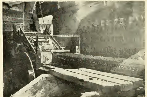
Extruding the clay column from the brick die
