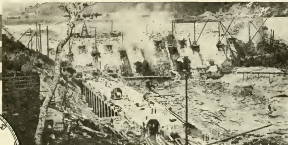
1902—Spier Falls Dam and Power Plant, Spier Falls, N. Y. Two #5 (2 yd) Ransome Mixers used.
