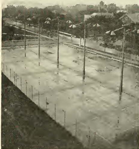
The new concrete tennis courts near the library. Note the overhead lighting system
