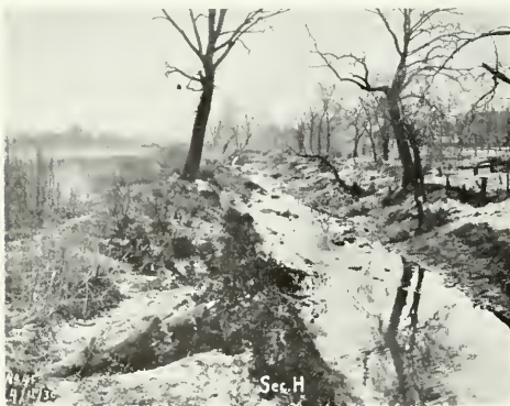
View of the River Des Peres during dry weather. Clearing of trees and underbrush on the right-of-way has been started, but the stream bed is in its natural condition.
