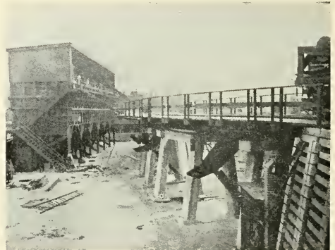
Figure 4: New coal yard served by the Illinois Terminal
