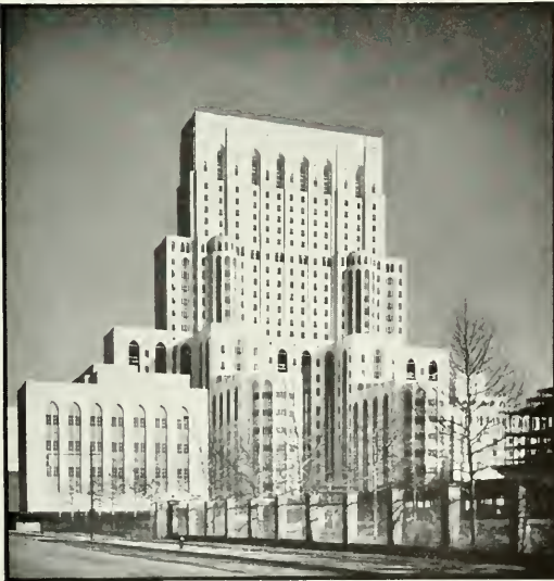
New York Hospital, Cornell Medical College. Jenkins valves serve plumbing, heating, power, in this great hospital . . . Jenkins Bros., 80 White St., New York, N. Y.; 510 Main St., Bridgeport, Conn.; 524 Atlantic Ave., Boston, Mass.; 133 N. 7th St., Philadelphia, Pa.; 646 Wash. Blvd., Chicago, Ill.; 1121 N. San Jacinto, Houston, Texas.
