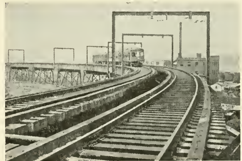
Figure 2: A portion of the elevated structure
