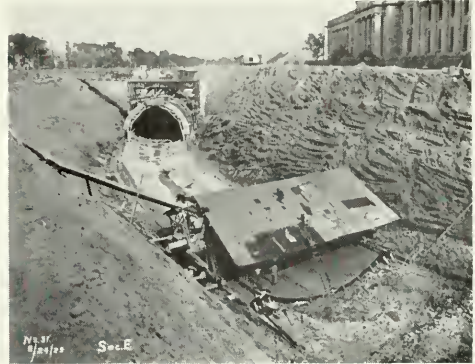
Construction of the 32-foot arch in front of the Jefferson memorial in Forest park at De Baliviere avenue
