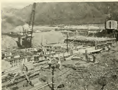
Caissons in the making
