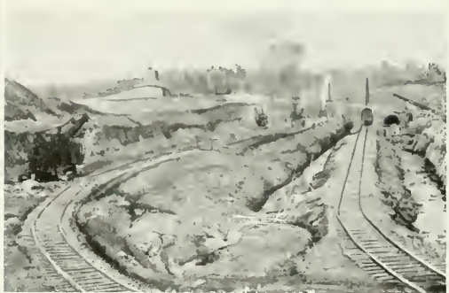
During the early stages of the excavation for the penstocks
