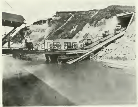
Incline and cradle, upper terminal at Memphis
