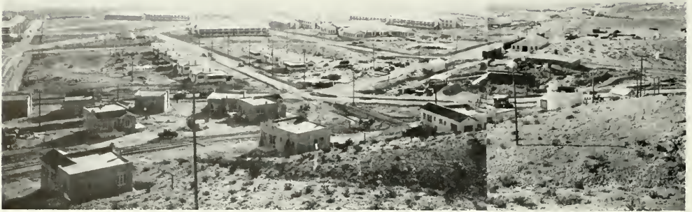
Panoramic view showing Boulder City, Nevada
