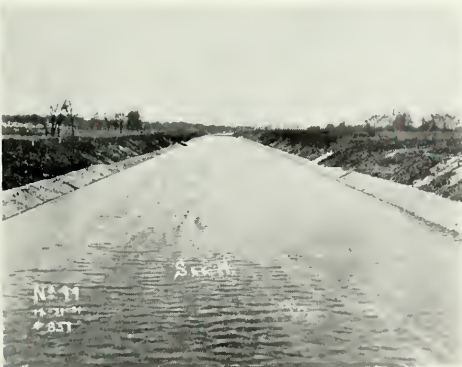
A view of section II flowing partially full. Notice the sewer outlet into the channel
