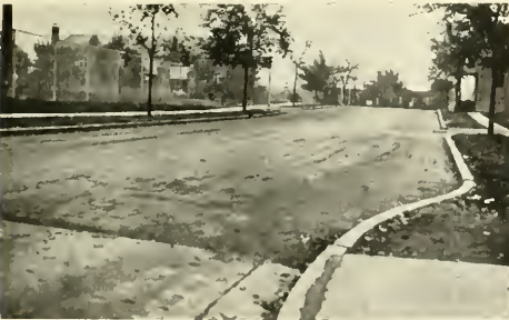
A view of the completed pavement on Sixth street, looking south from Armory avenue
