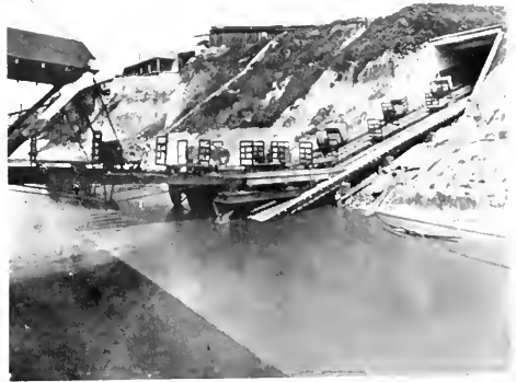
Incline and cradle, upper terminal at Memphis
