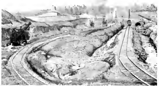
During the early stages of the excavation for the penstocks
