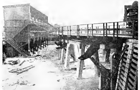
Figure 4: New coal yard served by the Illinois Terminal
