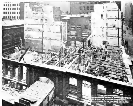
The Home Insurance building almost demolished, showing the skeleton framework used
