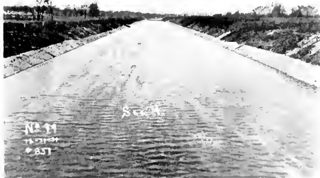
A view of section II flowing partially full. Notice the sewer outlet into the channel
