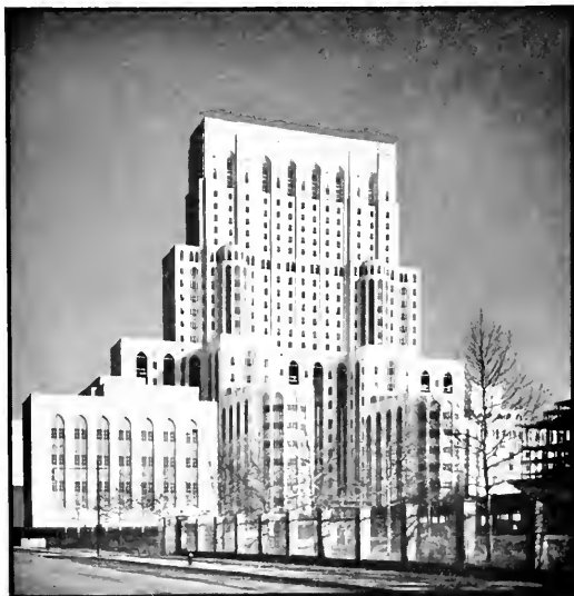
New York Hospital, Cornell Medical College. Jenkins valves serve plumbing, heating, power, in this great hospital . . . Jenkins Bros., 80 White St., New York, N. Y.; 510 Main St., Bridgeport, Conn.; 524 Atlantic Ave., Boston, Mass.; 133 N. 7th St., Philadelphia, Pa.; 646 Wash. Blvd., Chicago, Ill.; 1121 N. San Jacinto, Houston, Texas.
