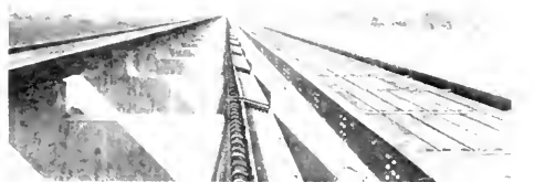
View from the top of the levees at Bonnet Carré
