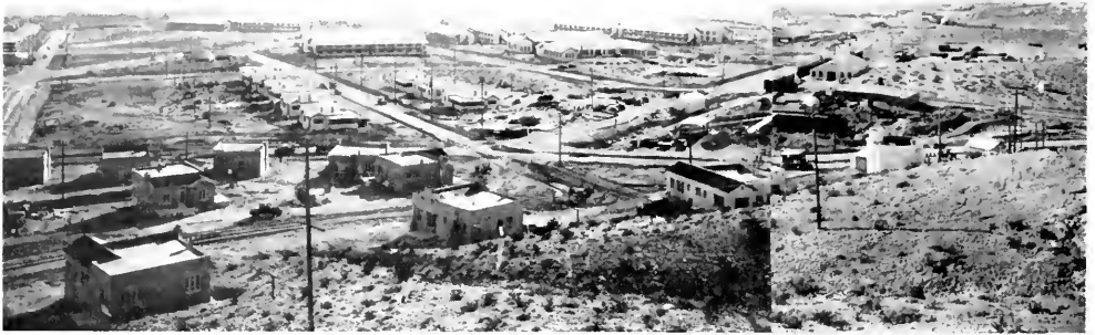
Panoramic view showing Boulder City, Nevada
