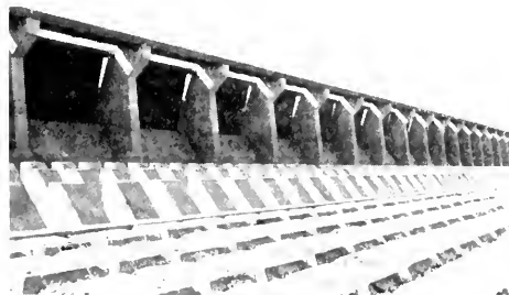
Downstream view of the Bonnet Carré spillway, showing the baffles and articulated slabs
