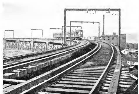
Figure 2: A portion of the elevated structure
