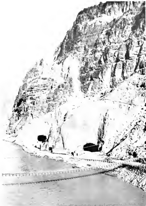
Upstream view showing tunnels on the Arizona side through which the Colorado river will be diverted during dam construction
