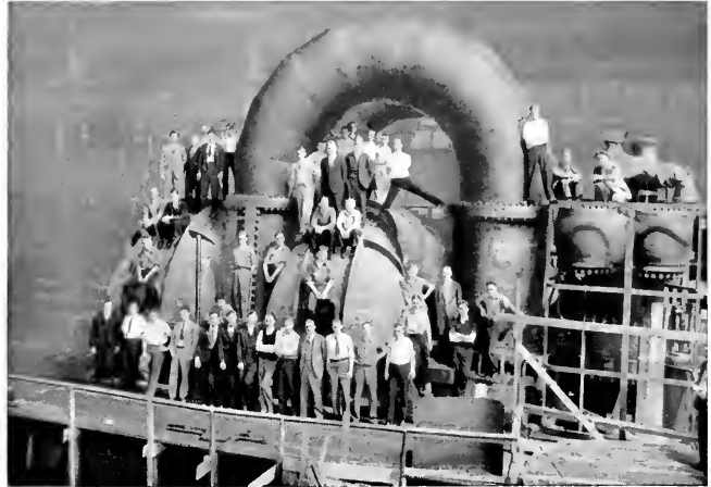
160,000-kw. G-E tandem-compound turbine-generator set on test.
