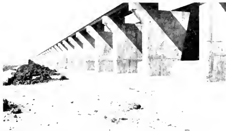
Upstream view of spillway of Bonnet Carré spillway. About 250,000 second-feet is to flow over this spillway into Lake Pontchartrain at flood time.
