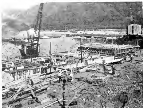
Caissons in the making
