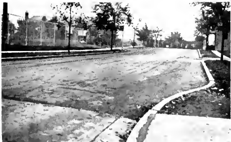
A view of the completed pavement on Sixth street, looking south from Armory avenue
