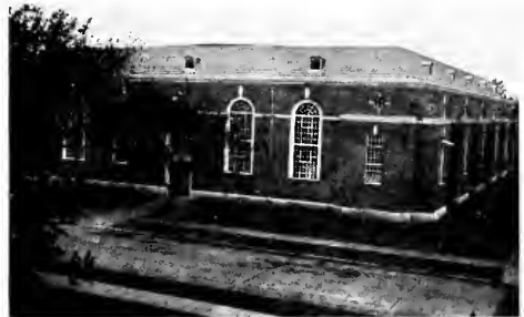
The completed skating rink, as seen from the armory
