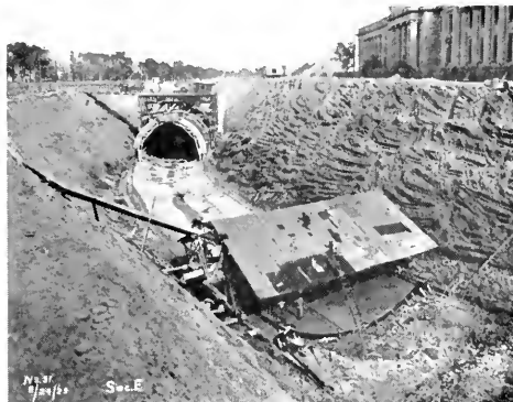
Construction of the 32-foot arch in front of the Jefferson memorial in Forest park at De Baliviere avenue
