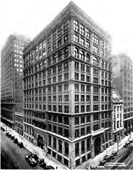
The Home Insurance building, Chicago, as it appeared before razing operations were started.
