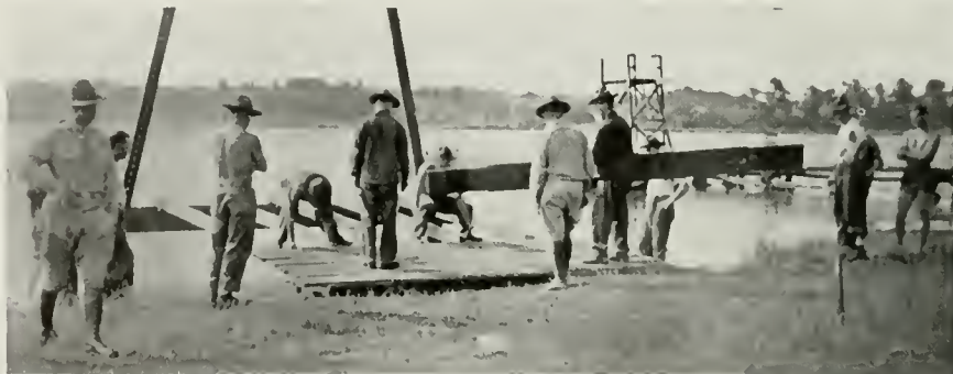
Student officers getting practical military bridge building experience.
