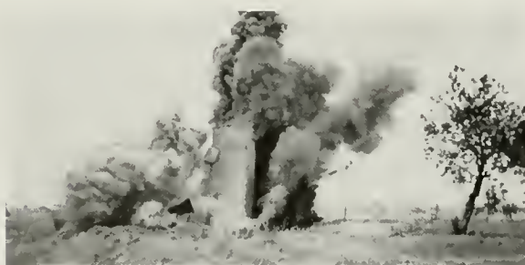
Engineers blowing down a silo at Camp Custer with T. N. T.
