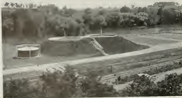
Sewage Sludge Digestors and Gas Holder, Janesville, Wis.
