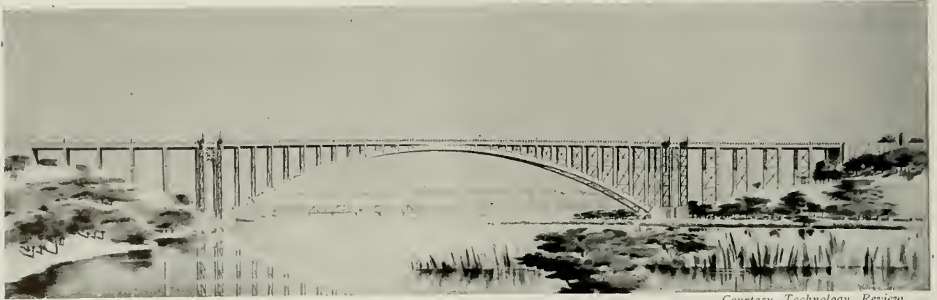
Largest Hingeless, Box-Girder, Single-Arch Span in the World—Hendrik Hudson Memorial Bridge, New York City
