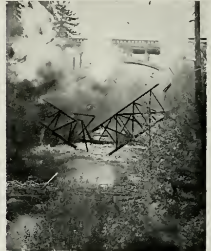
—Courtesy Engineering News-Record Clearing the Way
