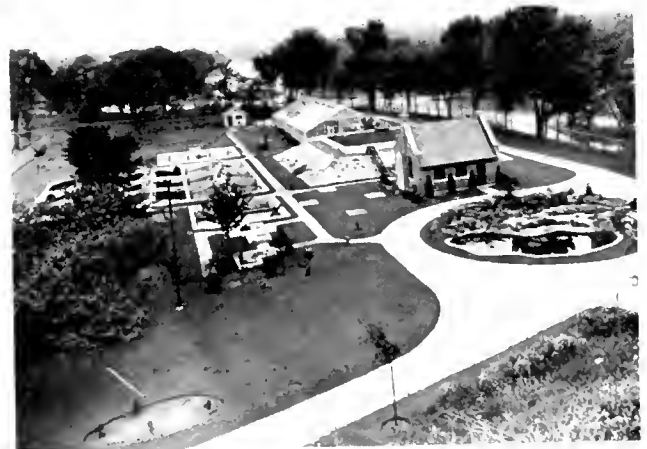
Attractive Sewage Treatment Plant at Geneva, Ill.
