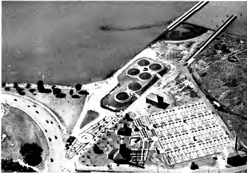
Airplane View of Westerly Sewage Treatment Plant at Cleveland, O.
