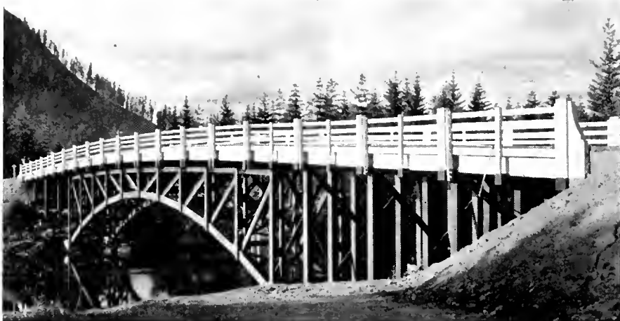
Three-Hinged Wood Arch Bridge
