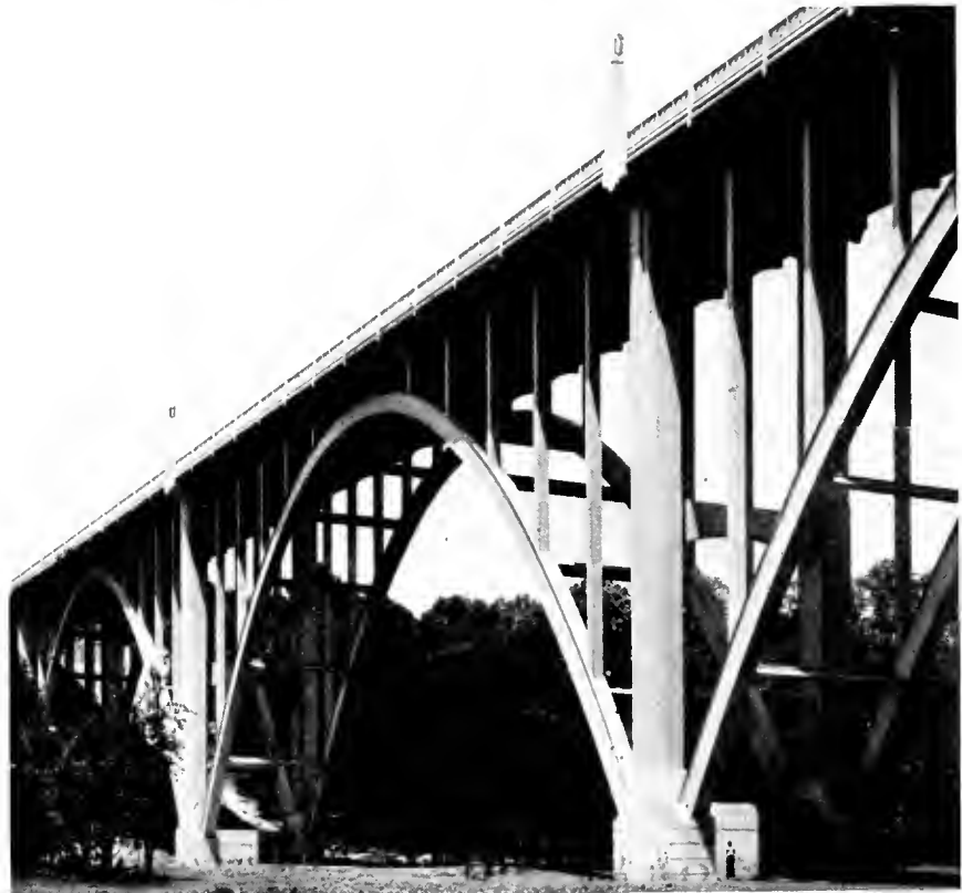
Grace and beauty are pronounced by the lines of the Lorain Road Viaduct in Cleveland.
