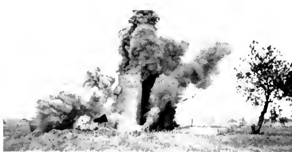
Engineers blowing down a silo at Camp Custer with T. N. T.
