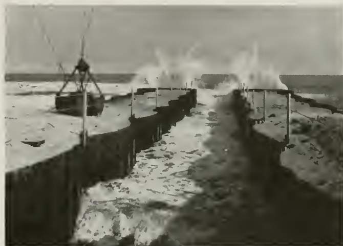
SEA WATER INTAKE
