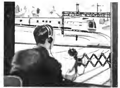
3. You ride more safely on the nation's railroads because of Western Electric train dispatching telephone equipment.
