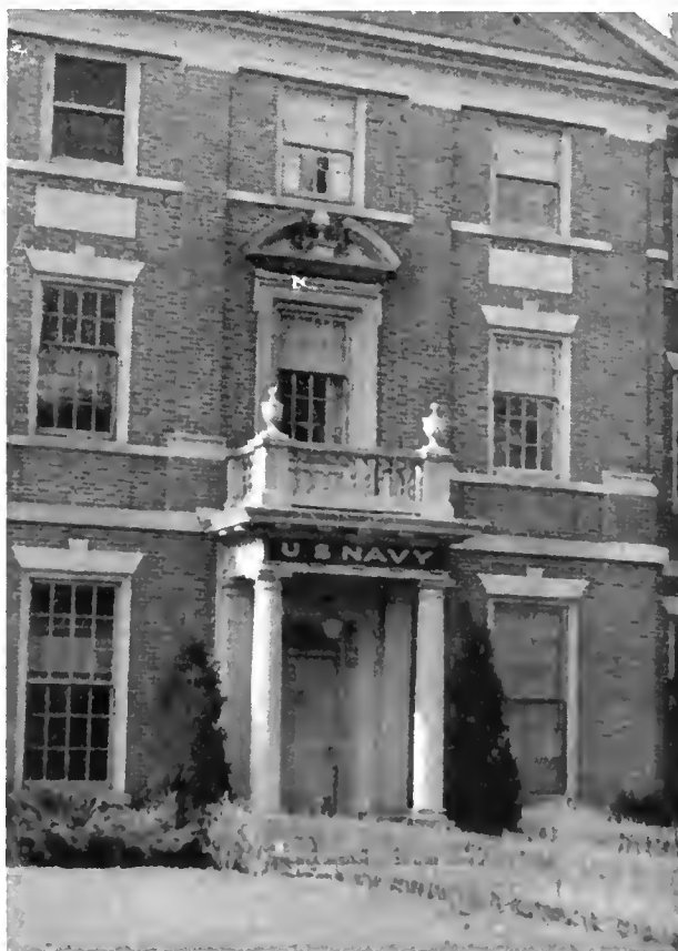
Main Entrance, V-12 Dormitories
