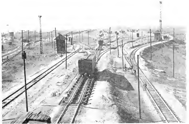
This is the Willis Hump Yard located in Galesburg, Illinois. The Yard is capable of handling approximately 80 to 95 trains in a 24-hour period and holds a record of 1,387 cars humped in an 8-hour period.
