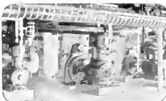
Three Frick Ammonia Compressors Give Dependable Refrigeration
