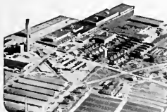
Air View of the Great Plant near Bridgeton, N. J.
