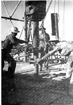
Two "tong men" breaking the drill-stem joint to add another section on the stem
