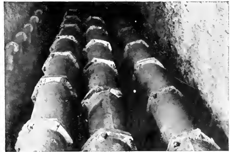
Section of 285-year-old cast iron water main still serving the town and fountains of Versailles, France.
