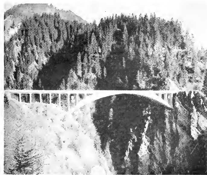
Maillart's bridges spring out of shapeless crags with the serene inevitability of Greek temples. Witness his Salginatobel bridge. (Photo from Giedion's "Space, Time, and Architecture.")
