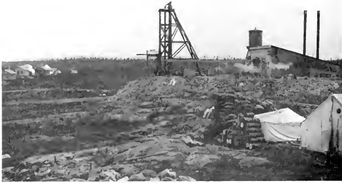
Equipment for the head frame of the God's Lake Mining Co. in Manitoba had to be shipped in by tractor over the winter ice roads.
