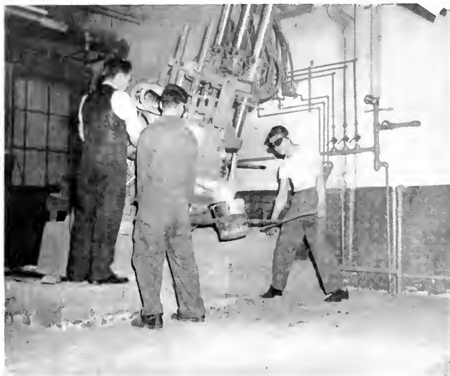
Electric arc furnace just installed at Navy Pier
