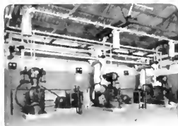
Three Frick Compressors under Automatic Control
