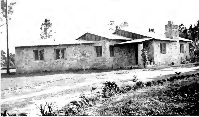
A typical example of what can be done by the use of rammed-earth construction methods. The house shown can be built at a much lower cost than would be possible with ordinary construction methods.
