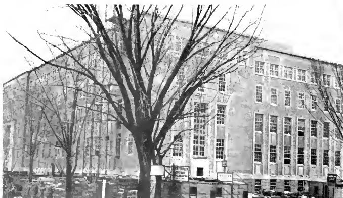
The new Chemistry and Chemical Engineering building at the corner of Matthews and California streets is nearing completion. Photo by Al Augustyn.)
