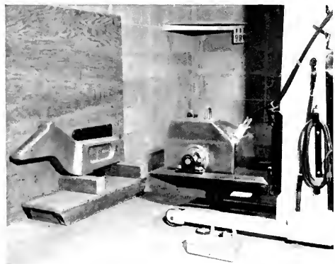
Ripper shank being radiographed with cobalt 60 projector
