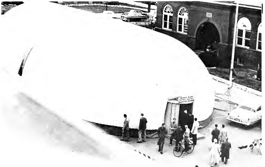
This air tent will house all the Agricultural Engineering displays. It is supported by air blown from a crop dryer.
