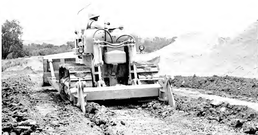
Caterpillar D8 Tractor with ripper tearing through road material
