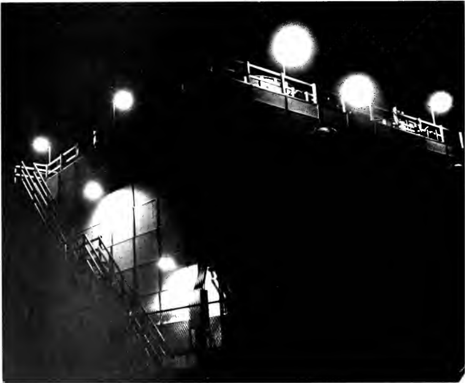
POWER PLANT (M.E. 263 PROVING GROUND)
