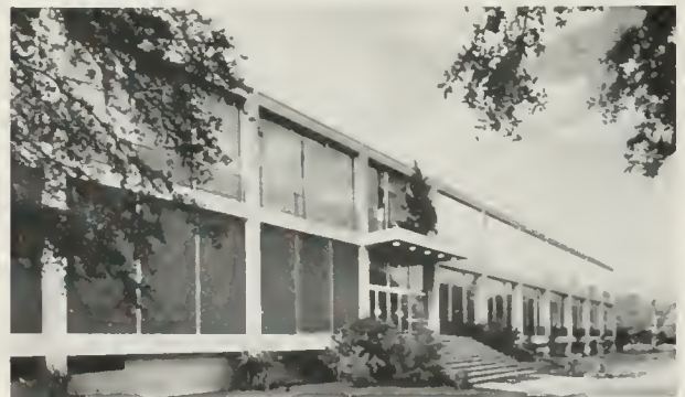
UNIVERSITY CENTER features swimming pool, bowling lanes, radio station, cafeteria, ballroom. MAIN ARCHITECTS: Curtis & Davis and Associates; Edward Silverstein. GENERAL CONTRACTOR: Farnsworth & Chambers. MECHANICAL CONTRACTOR: Sciambra & Masino. CONSULTING ENGINEERS: Leo S. Weil; Walter B. Moses.
