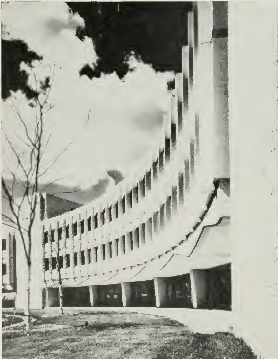
The new General Offices Building of the American Baptist Convention, Valley Forge, Pa.
