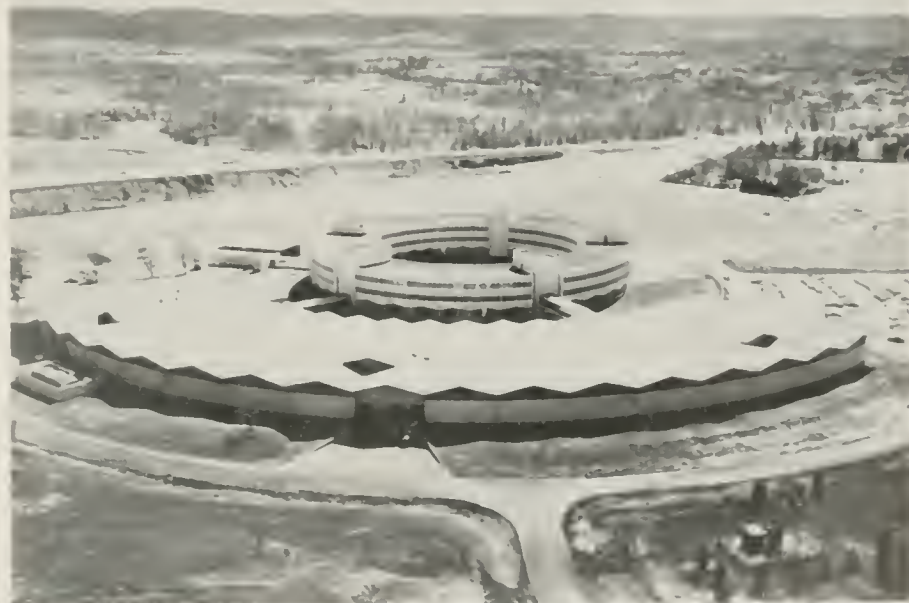
The 240 feet inner diameter and 52 feet width of the office building provides offices free of any wedge-shaped feeling and a convenient partitioning module.
