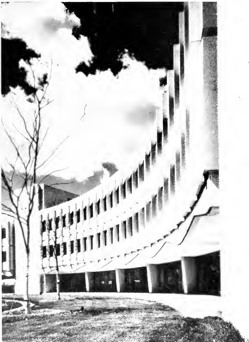
The new General Offices Building of the American Baptist Convention, Valley Forge, Pa.
