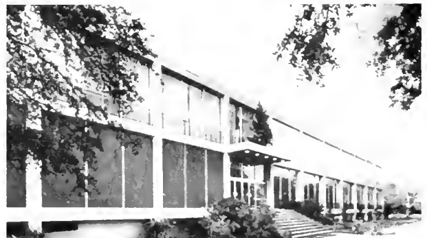
UNIVERSITY CENTER features swimming pool, bowling lanes, radio station, cafeteria, ballroom. MAIN ARCHITECTS: Curtis & Davis and Associates; Edward Silverstein. GENERAL CONTRACTOR: Farnsworth & Chambers. MECHANICAL CONTRACTOR: Sciambra & Masino. CONSULTING ENGINEERS: Leo S. Weil; Walter B. Moses.
