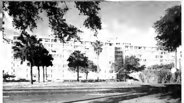
APARTMENT BUILDING for married students. MAIN ARCHITECTS: Goldstein, Parham & Labouisse. GENERAL CONTRACTOR: J. A. Jones Construction Co. MECHANICAL CONTRACTOR: Sciambra & Masino. PLUMBING CONTRACTOR: Jas. F. O'Neil Co., Inc. CONSULTING ENGINEERS: Design Engineers & Associates.
