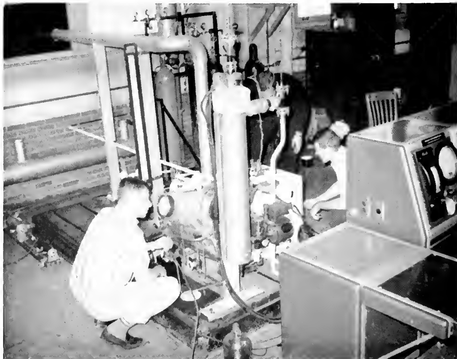
Figure 1. As part of the practical application of the theory taught in the classroom, several Mechanical and Industrial engineering students are shown running tests on the adiabatic compression machine in the Internal Combustion Engine Laboratory.
