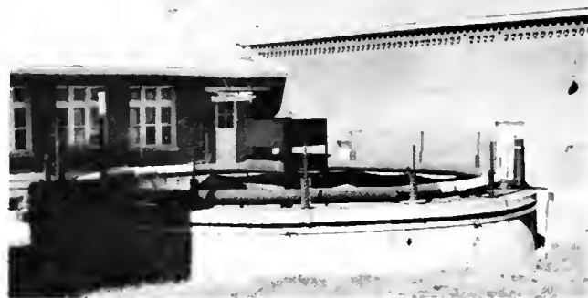
This circular concrete casing can be found just east of the Electrical Engineering Research Laboratory, and on the north bank of the Boneyard.
