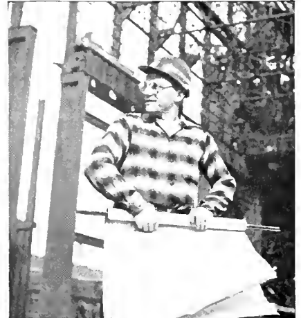
DON DIXON, C.E., MASSACHUSETTS '60 —A field engineer in our Fabricated Steel Construction Division, Don supervises steel erection for major buildings and bridges.
