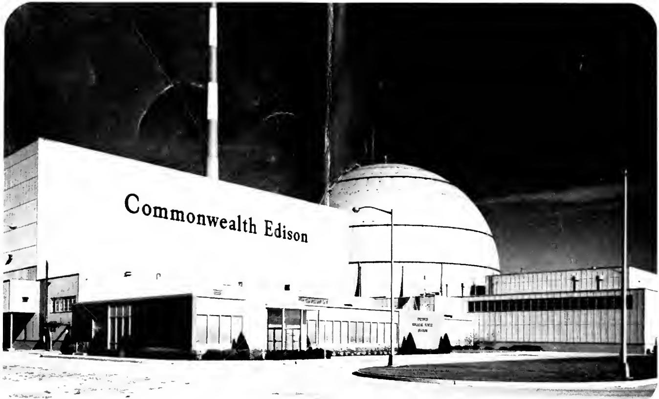
DRESDEN NUCLEAR POWER STATION —America's first full-scale producer of commercial electric power from the atom, rated 200,000 kw.
