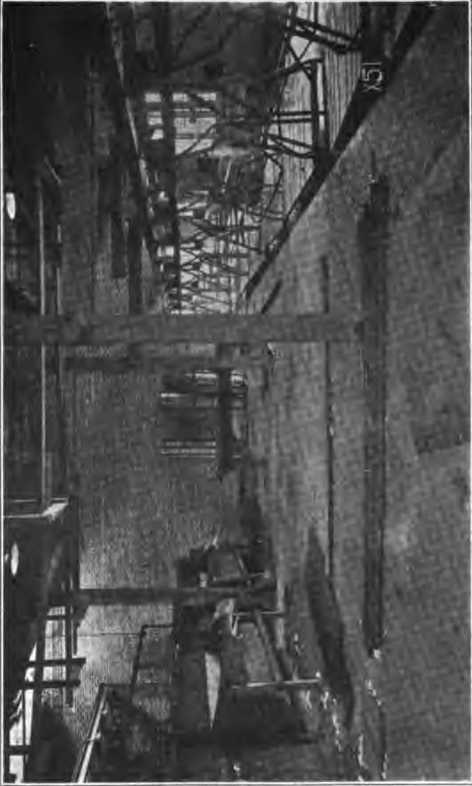
FIG. 25.—COTTON DRY HOUSE, SHOWING DELIVERY APRONS AT END OF DRYERS (E. I. DU PONT DE NEMOURS CO.)
