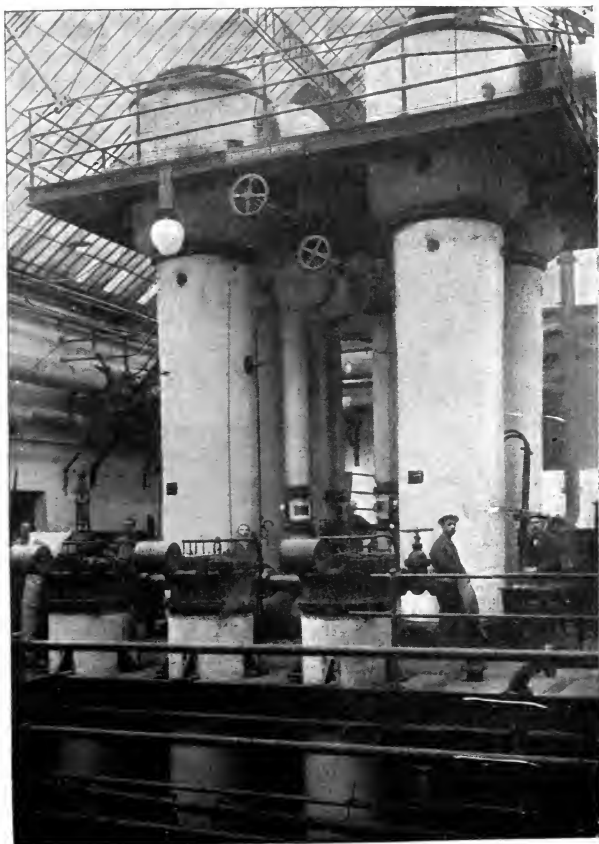
FIG. 223A.—Kestner quadruple effect. Tirlemont sugar refinery, Belgium.
