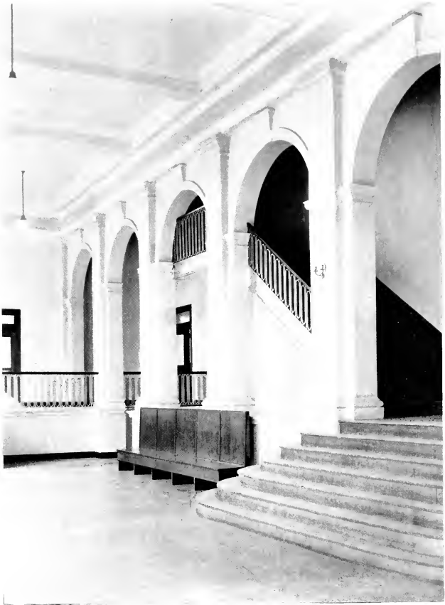
WRIGHT BUILDING LOBBY
