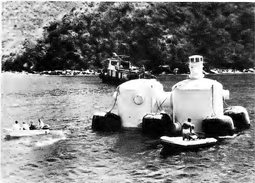
Figure 15. Habitat Moored at Ballasting Site Being Supported by Six 8,8 Ton Salvage Pontoons
