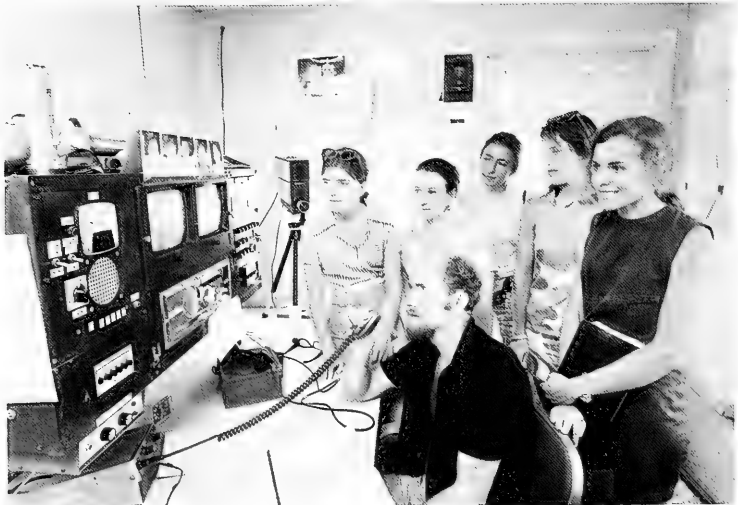
Figure 11. Command Van Control Console
