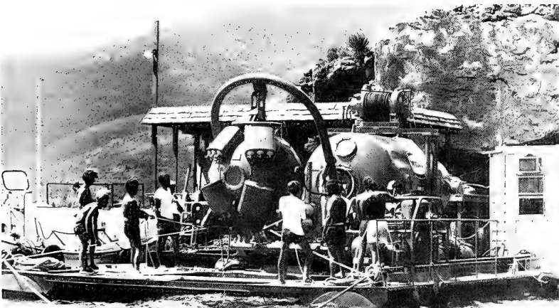
Figure 5. The Barge-Mounted Decompression Facility Moored Adjacent to the Dive Platform. The surface support center is shown in the top center of the Photograph.
