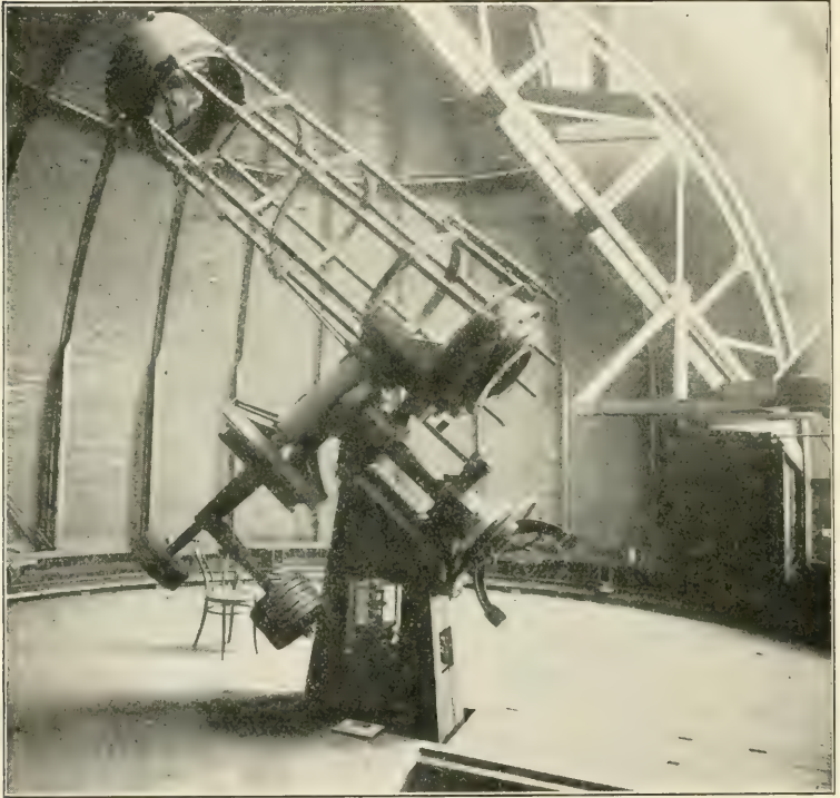
FIG. 32.—Reflector with Skeleton Tube (Brashear).
