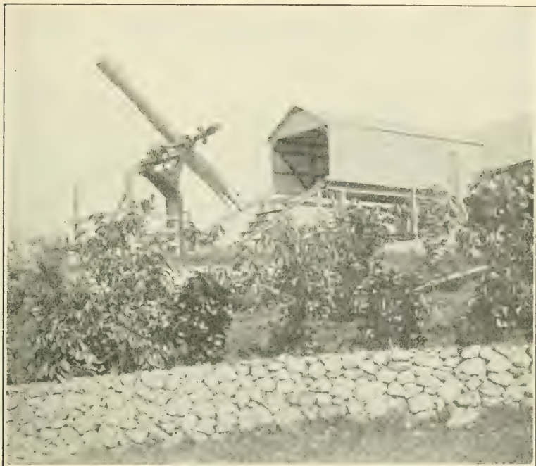
FIG. 175.—Sliding Housing for 11-inch Refractor.
