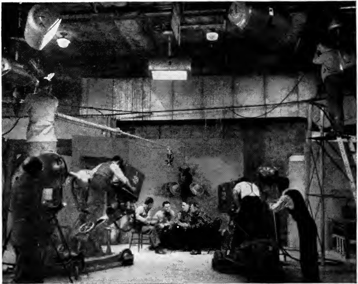
FIG. 36.—Mercury-vapor water-cooled ceiling lights in use in studio of WRGB, General Electric's television station. Floor lamp of same variety is visible, too. ( General Electric Company. )
