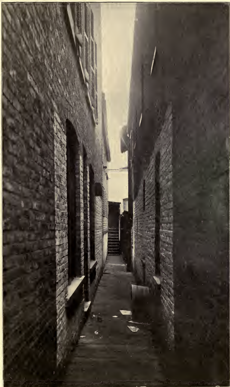
HOUSES COVERING ALL OF LOT
