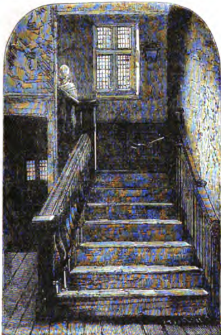
OLD STAIRCASE IN THE RESIDENCE OF DR. JOHNSON.
