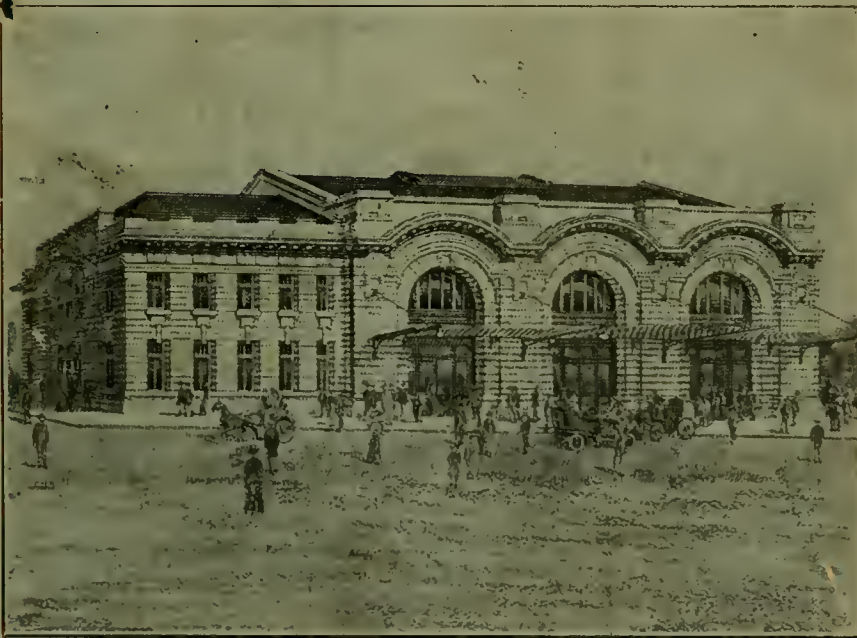
MUNICIPAL BUILDING. UNDER CONSTRUCTION
