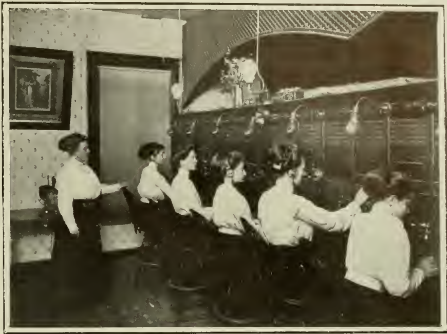
SWITCH BOARD OF RALEIGH TELEPHONE COMPANY Inc.
