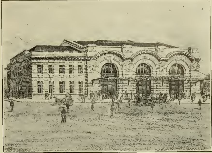
MUNICIPAL BUILDING. NOW UNDER CONSTRUCTION
