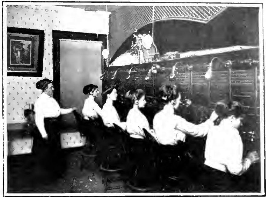
SWITCH BOARD OF RALEIGH TELEPHONE COMPANY Inc.
