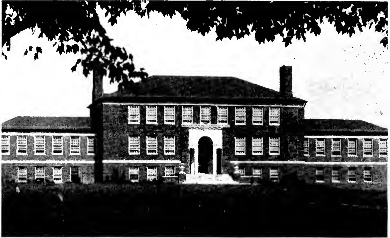
HORT BUILDING, A STRUCTURE A CAMERA NEVER DOES JUSTICE
