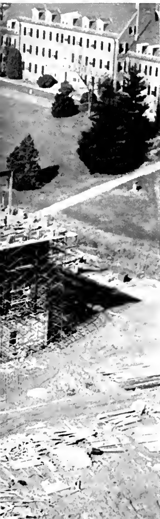
CONSTRUCTION ELEVATOR towers over scaffolded stack walls facing Annie A. ▶
