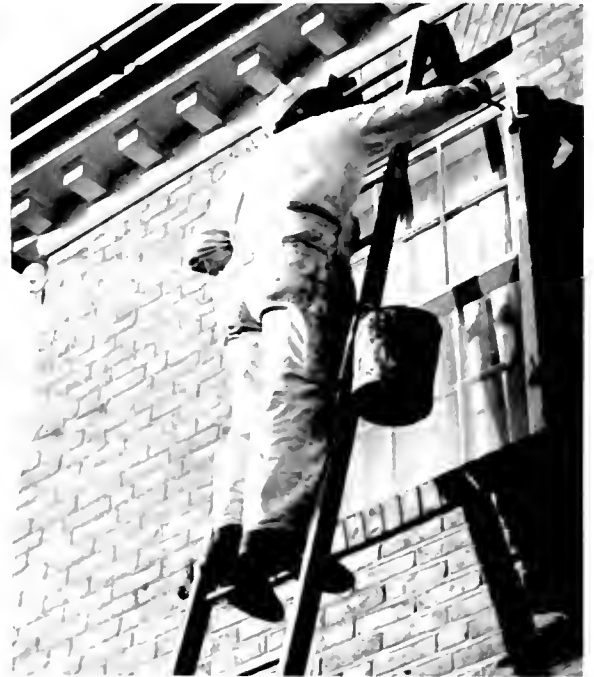
PAINTER puts finishing touches on bedroom window.
