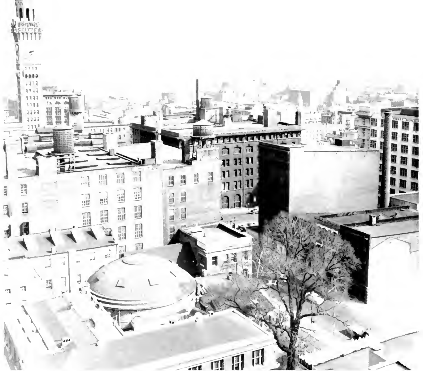
VIEW EASTWARD FROM TOP OF HOSPITAL SHOWS OLDER BUILDINGS—DOMED MED SCHOOL, AD BUILDING, RESEARCH LABORATORY.
