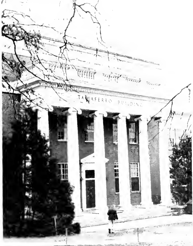
TALIAFERRO BUILDING . . . home of the College of Business and Public Administration.
