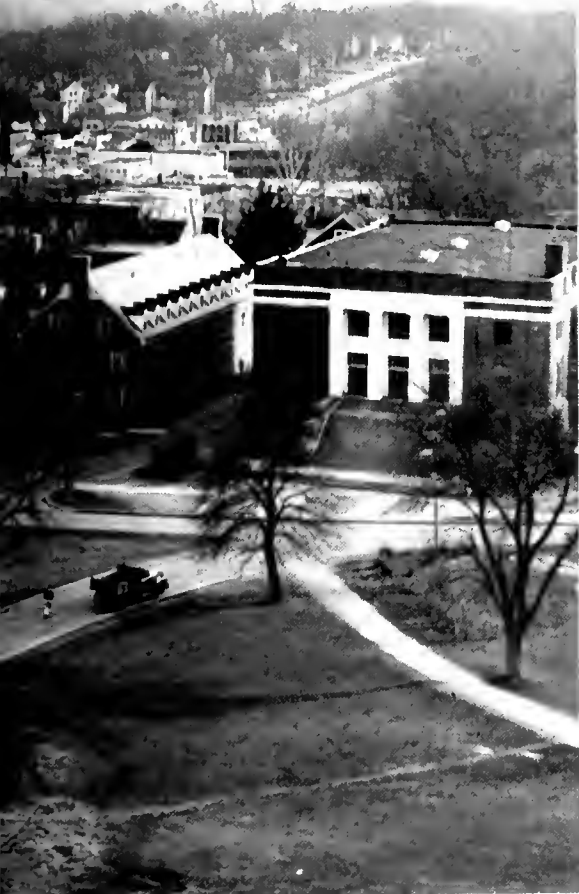
COLLEGE PARK panorama surrounds Montgomery Hall as seen from Chapel steeple.
