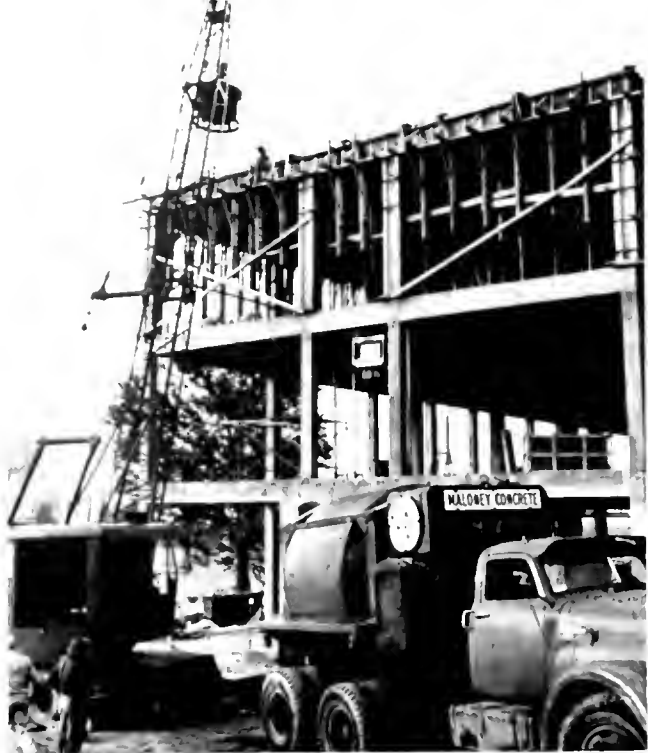
IN CONSTRUCTION STAGES, Journalism Building looked like this last spring. Work got off to late start.
