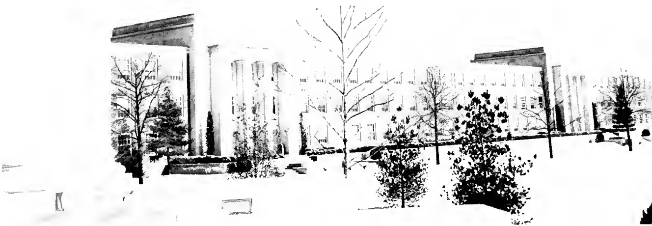
A WINTRY SETTING for the sleek lines of the Engineering Building.
