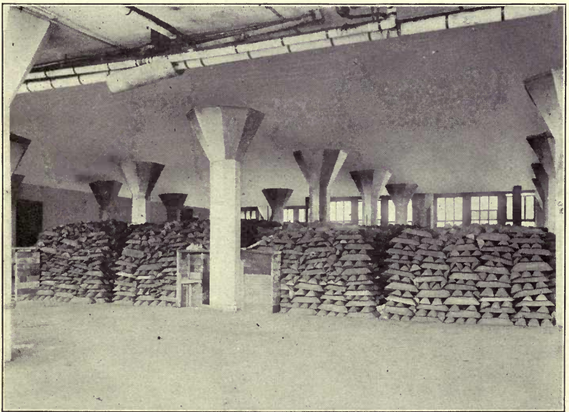
FIG. 2. VIEW SHOWING FULL LOAD ON FLOOR
