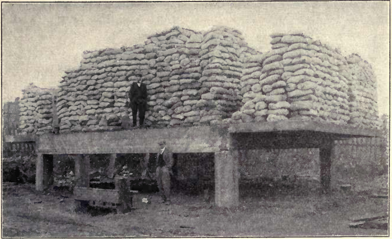
FIG. 9. BARR PANEL TEST; SAND IN SACKS AS A LOADING MATERIAL.
