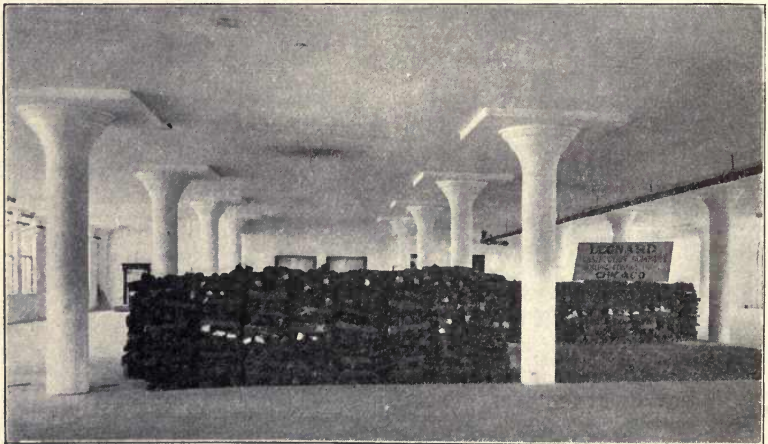
FIG. 10. FRANKS BUILDING TEST; PIG-IRON AS A LOADING MATERIAL.
