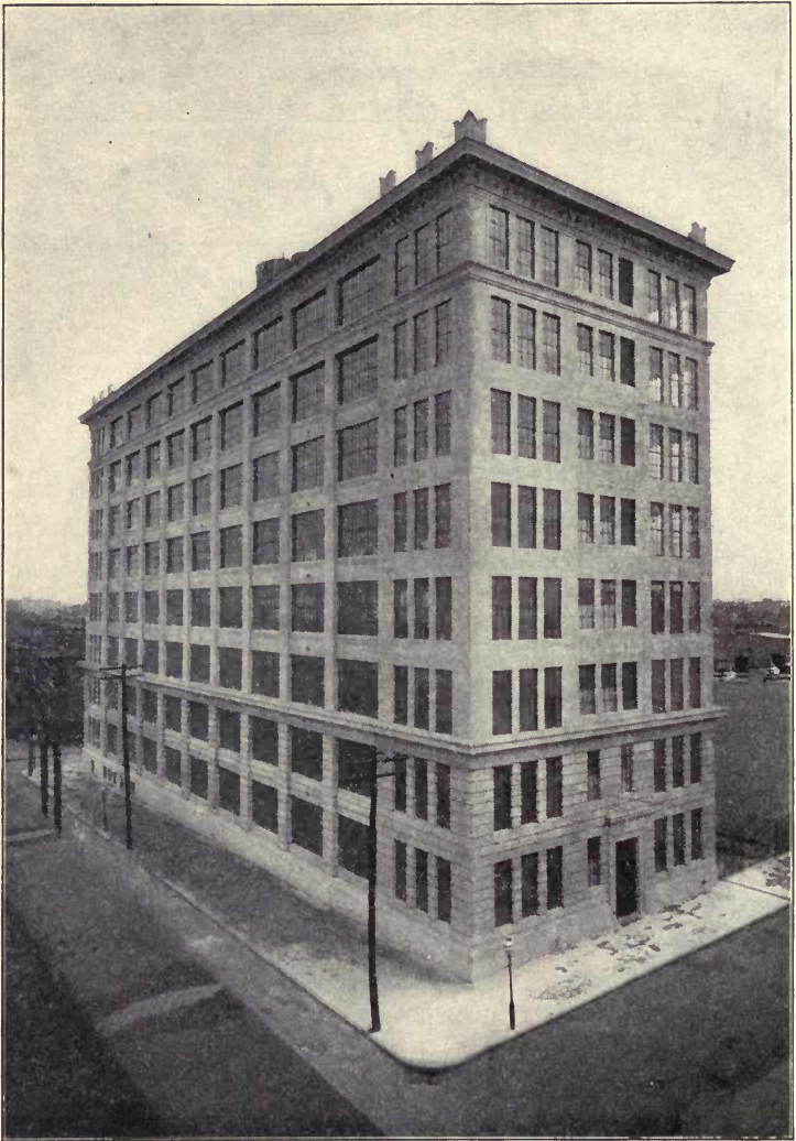
FIG. 40. THE TURNER-CARTER BUILDING.
