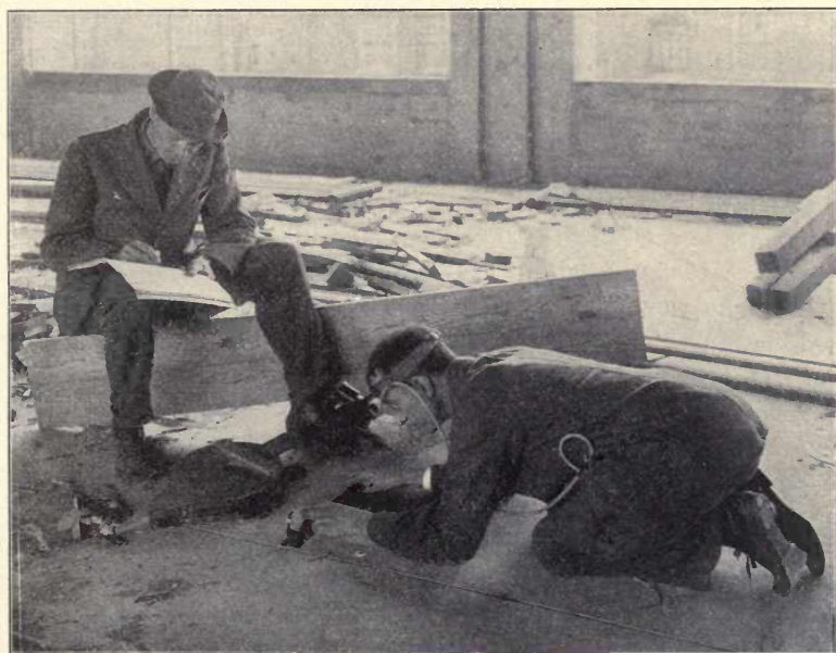
FIG. 16. TURNER-CARTER BUILDING TEST; TAKING AN OBSERVATION ON A STANDARD GAUGE LINE.
