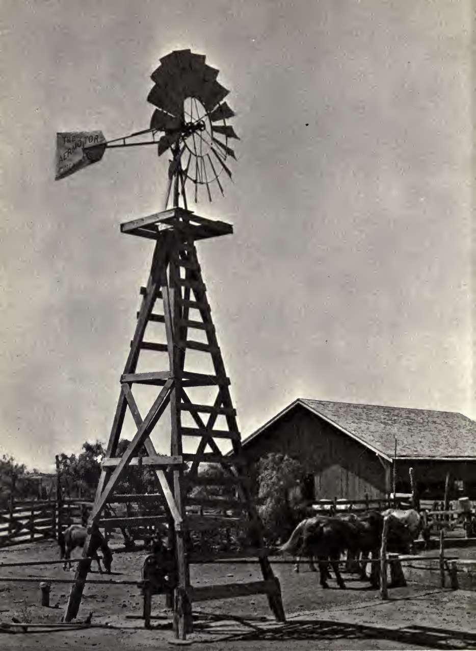
WINDMILL, WATERING TROUGH, AND BARN, NEAR SPUR
