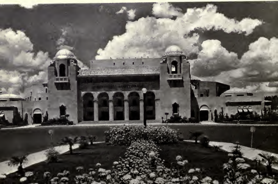
MUNICIPAL AUDITORIUM, SAN ANTONIO
