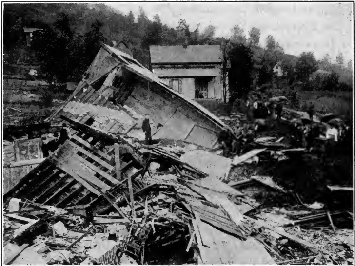
FIG. 48.—The effects of a tornado.
