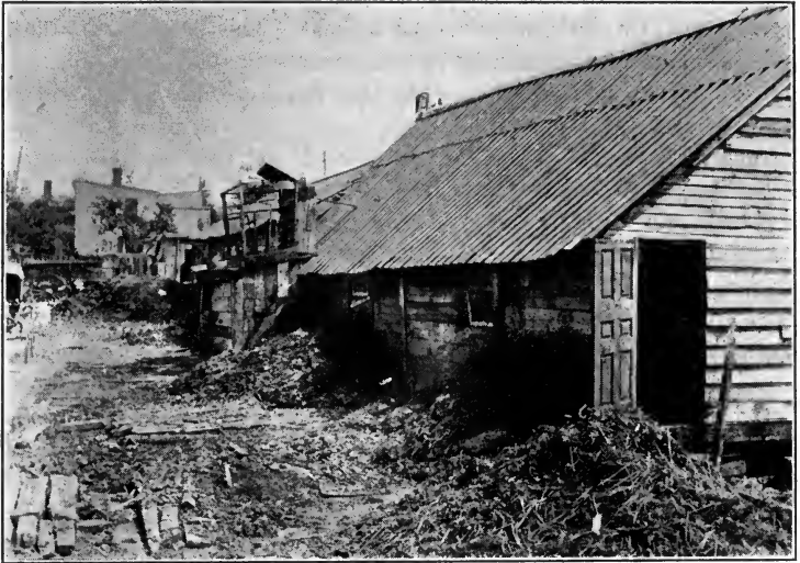
FIG. 18.—Insanitary conditions here.
