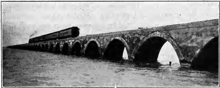
FIG. 62.—Concrete construction. (Courtesy of the East Florida Railway Company.)
