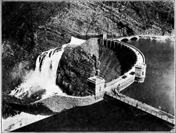
FIG. 38.—The Roosevelt Dam on Salt River, Arizona, is 280 feet high. It has a storage capacity sufficient to cover with water 1,367,000 acres one foot deep. Below the dam, and out of sight in the picture, is a power-house capable of developing 7,500 horsepower.
