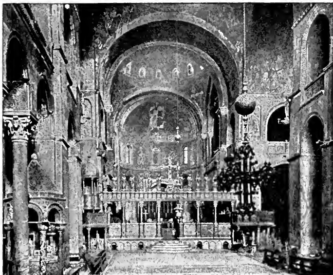
FIG. 80.—INTERIOR OF ST. MARK'S.
