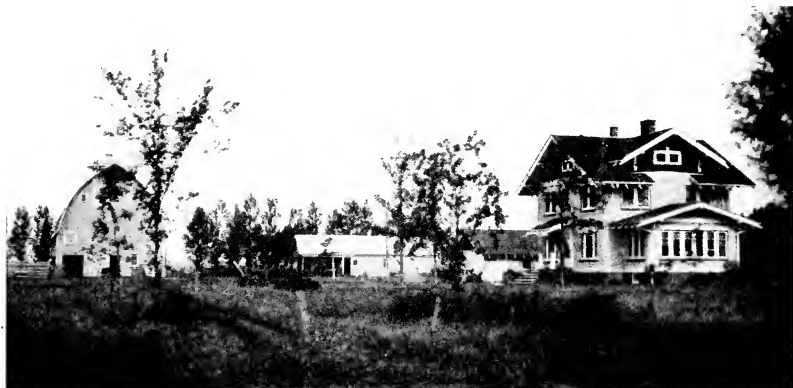
FIG. 81. VIEW FROM MAIN ENTRANCE
