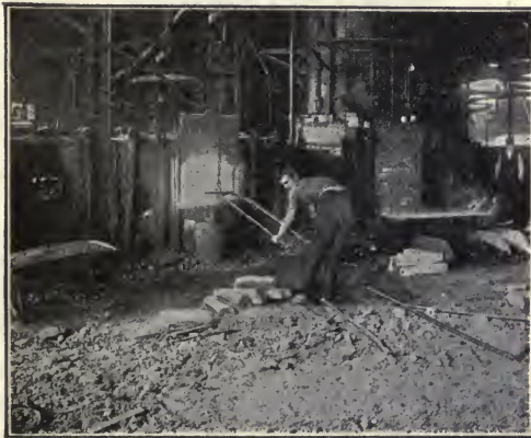
Courtesy of Interstate Iron and Steel Co.
