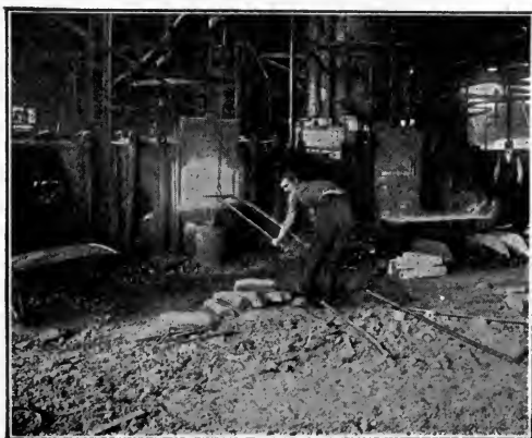
Courtesy of Interstate Iron and Steel Co.
