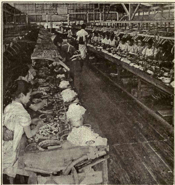
FIG. 65.—MODERN METHOD OF SOFTENING AND REELING SILK FROM COCOONS.
