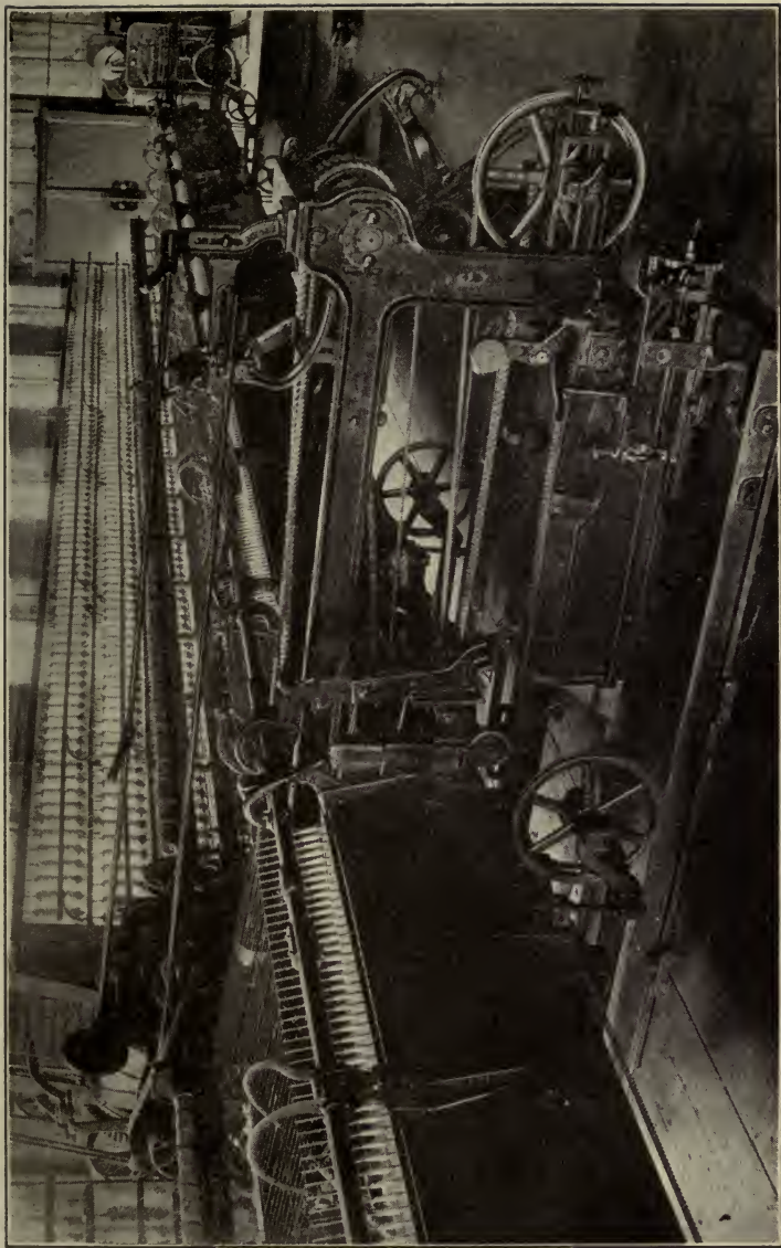
FIG. 22.— MULE SPINNING. Courtesy of the Mason Machine Works.
