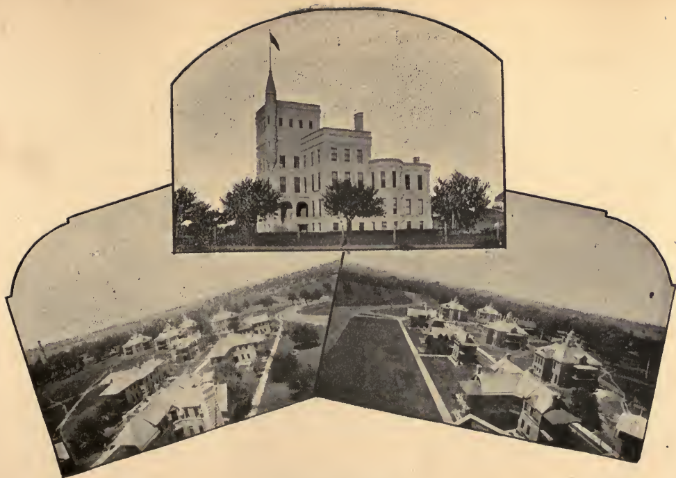
Headquarters Building. Illinois State Soldiers' and Sailors' Home.
