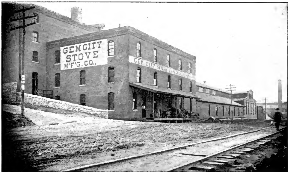
Gem City Stove Manufacturing Company.
