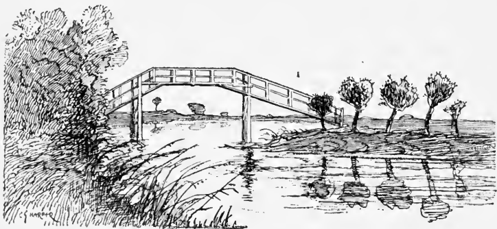
WOODEN BRIDGE ACROSS THE UPPER THAMES.
