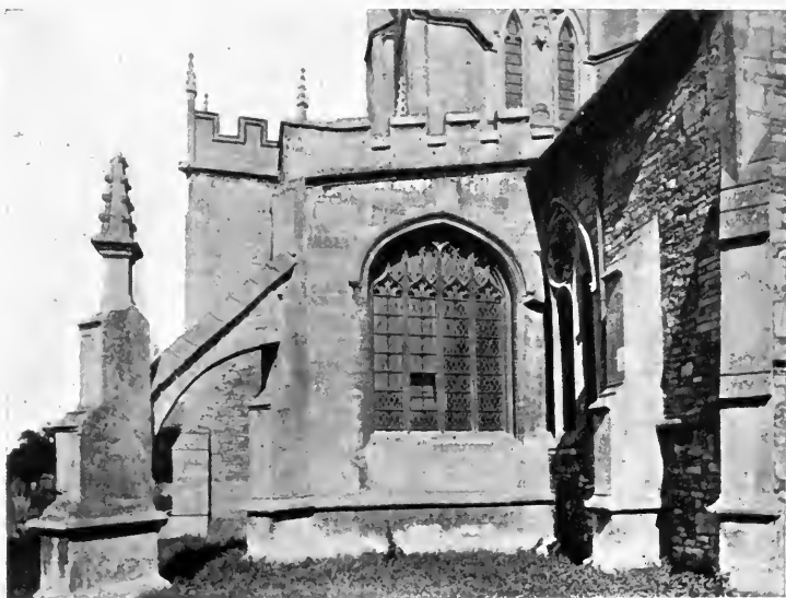
STRAINER-BUTTRESS, ST. SAMPSON'S, CRICKLADE.
