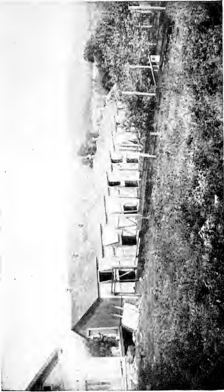
The henery is 150 feet long and 15 feet wide, divided into ten sections
